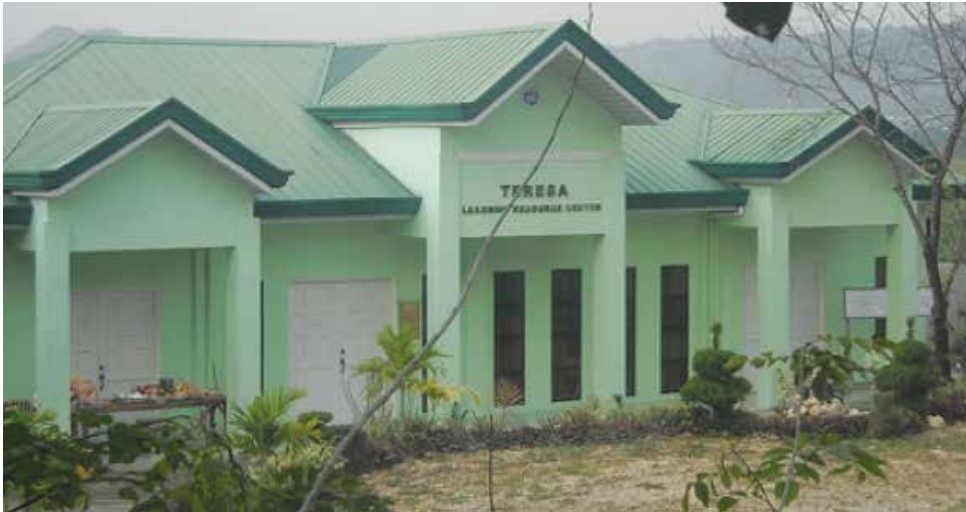
The Integrated Solid Waste Management Facility in Teresa, Philippines operates a Learning Resource Center where waste management training is offered to local government units and interested parties for a fee. Photo credit: Teresa Municipal Environment and Natural Resources Office
