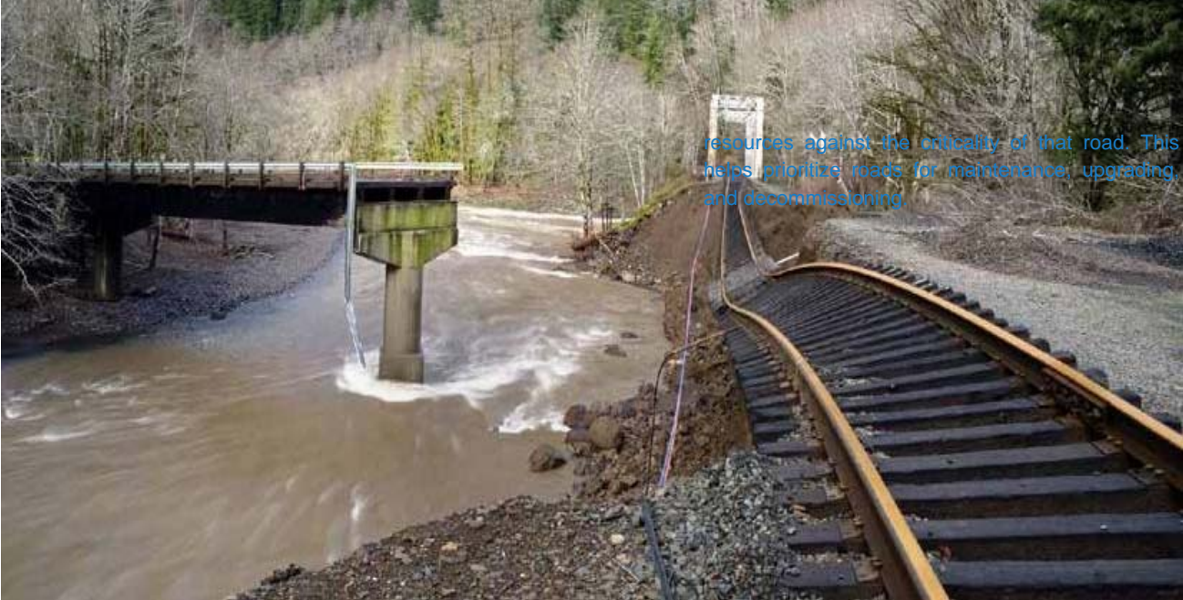
Salmonberry Bridge & Port of Tillamook Bay Railroad damaged during the Dec. 3, 2007, flood. Lower Nehalem River Road Confluence of the Salmonberry River & the Nehalem River, Salmonberry Oregon.
