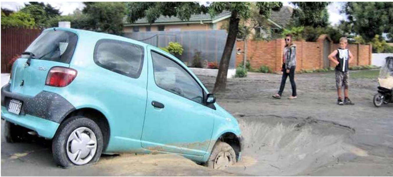
Sinkholes and Liquefaction North New Brighton in Christchurch
