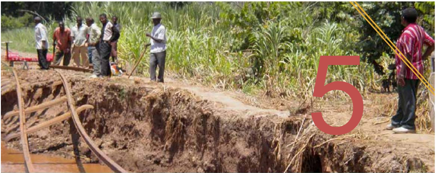
A U.S. Army Africa engineer views Tanzania flood damage in 2010.
