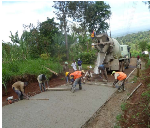
Rural concrete slabs undertaken as part of Dfid's AFCAP (African Community Access Programme). Source: Roughton
