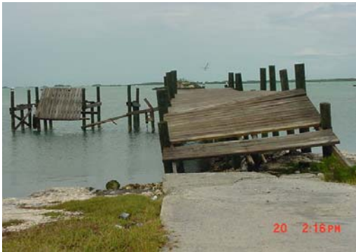
Photos: Bahamas Timber Jetties, after Hurricane Floyd: Source: IMC Worldwide
