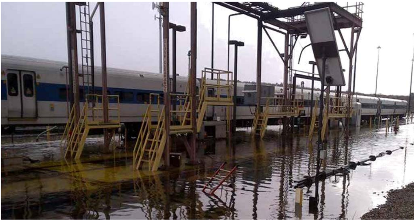
Flooding and damage to Metro-North's system—in the aftermath of Hurricane Sandy—to the bridge and south yard at Harmon.
