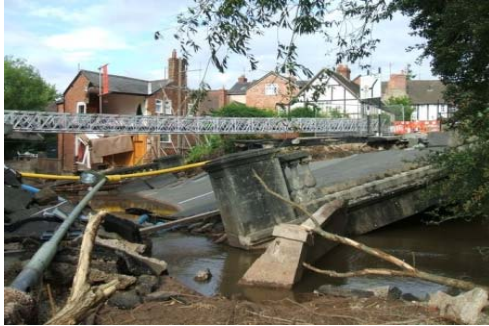
Flood Damage Burway Bridge over the River Corve after the floods (UK). Source: DI Wyman and is licensed for reuse under the Creative Commons Attribution-Share Alike 2.0 license . Date 3 July 2007
