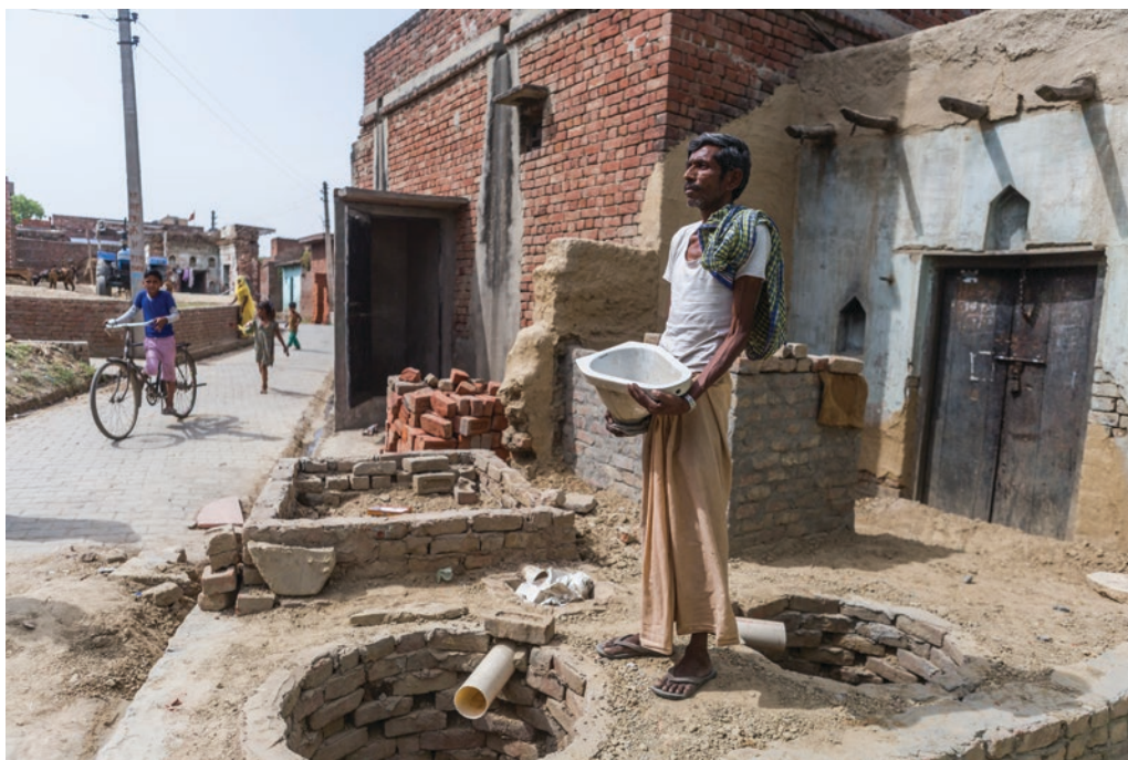
PHOTOGRAPH 12.1. Twin Pit Latrine Construction
