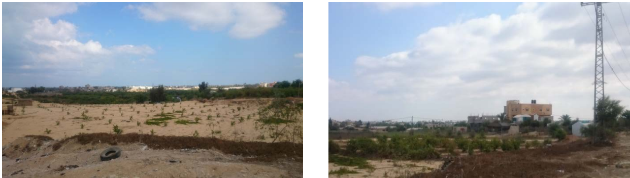
Figure 5-9: Photos for the proposed location of the Main Pumping Station (GVC/CEC, October, 2017)
