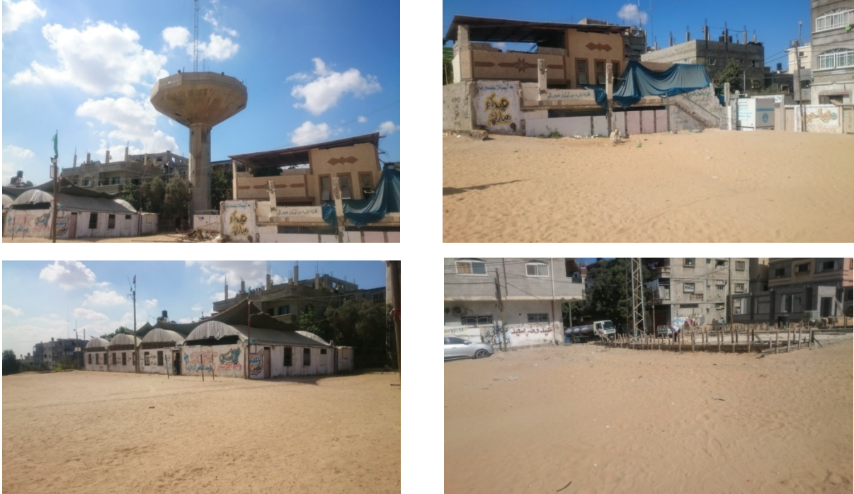
Figure 5-12: Photos for the proposed location of the BL-T01 B Reservoir in Jabalia (GVC/CEC, September, 2017)
