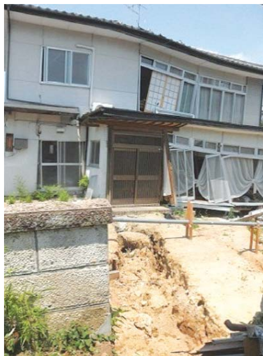
Figure 2.10 Houses damaged by failure of retaining walls
