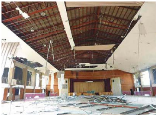
Figure 2.8 Fallen ceiling panels in school gymnasium
