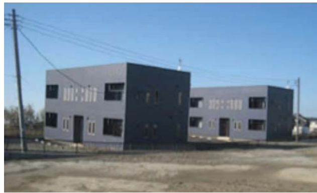
Figure 2.9 Subsidence of houses from liquefaction
