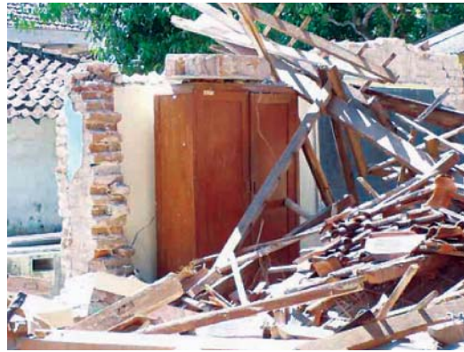
Figure 2.12 Collapsed school building in which furniture is still standing (Yogyakarta province, following Central Java Earthquake, 2006)
