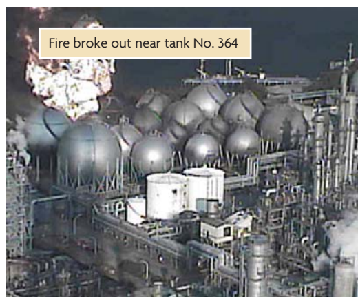
Figure 5.5 Leaked LPG catches fire at a refinery
