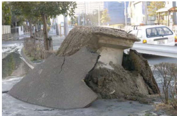
Figure 20.3 Manhole raised by liquefaction in Urayasu City
