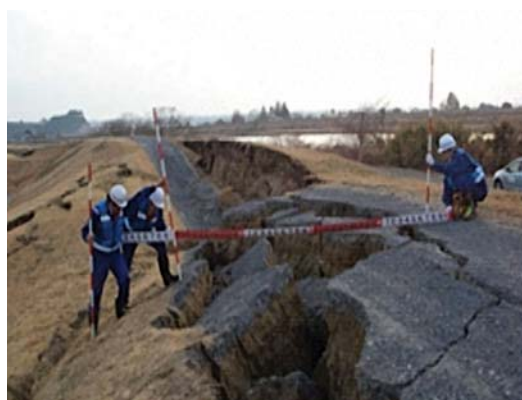
Figure 3.2 Damage to river dikes at Narusegawa
