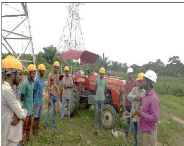
Figure 5.4 Use of Tractor for Stringing
