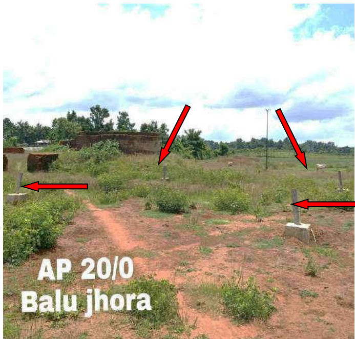
Tower footing of AP 20/0 (arrow)
