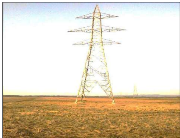
Figure 5.5 Construction during lean period
