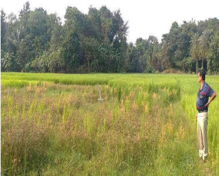
Visit of Tower location at AP 27/0 of 132 kV Phulbari- Ampati line
