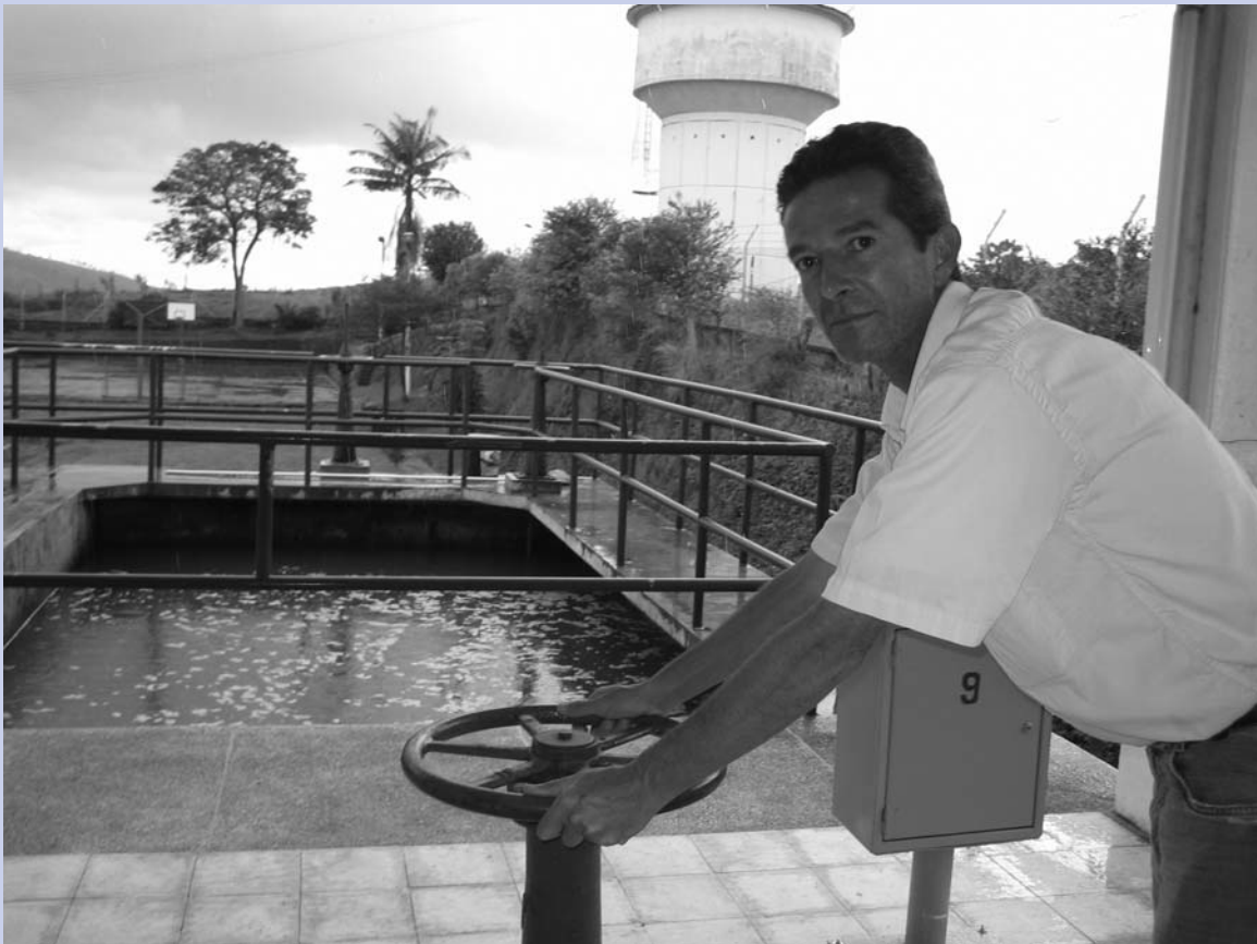
MDP-funded municipal water treatment plant in Pereira, Colombia. Photo courtesy of Roy Gilbert.
