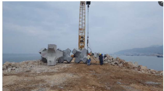
Protecting fishing port from storm surges
