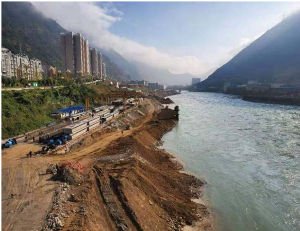
Flood prevention works under construction
