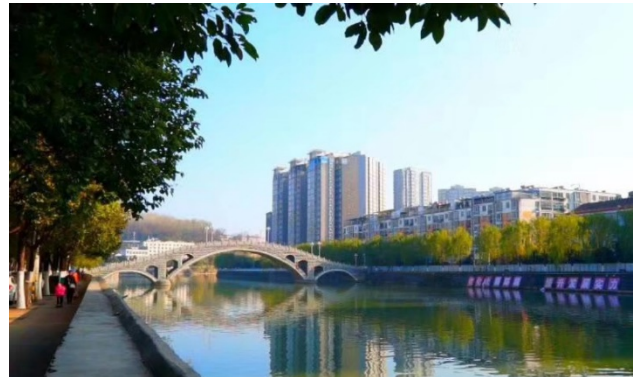
Urban flood management works
