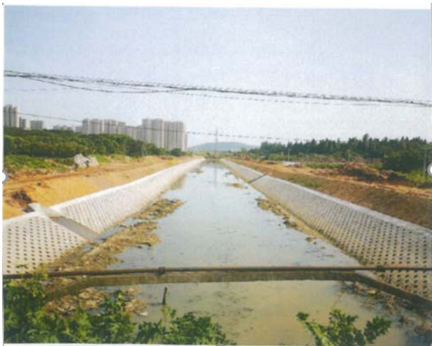
A tributary under rehabilitation
