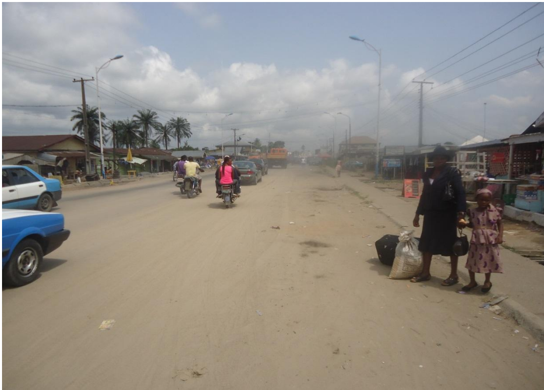
Plate 4.1: Accumulated Sand on Okirigwe Roundabout, Sapele, Delta State
