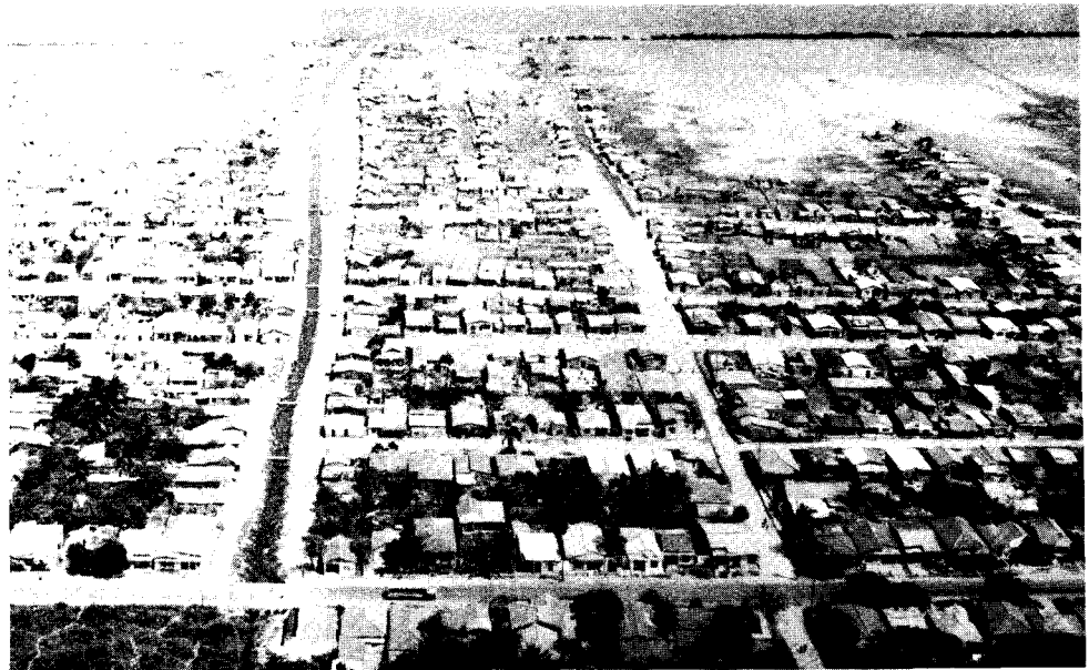
View of Tabu drainage ditch towards the Lagoon
