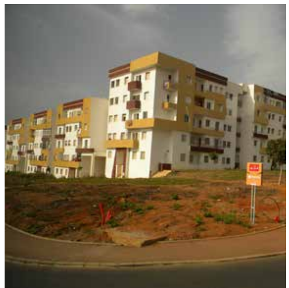
Housing units in Rabat, Morocco © UN-Habitat
