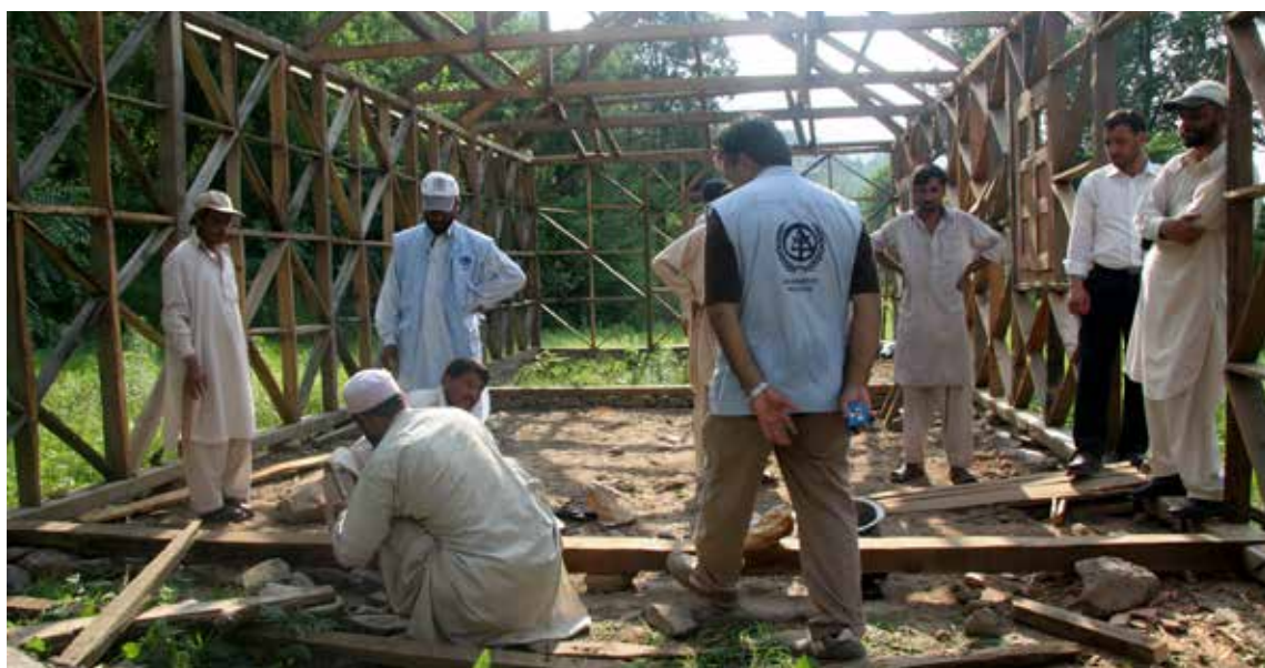
Reconstruction of a house in Bagh, Pakistan © UN-Habitat
