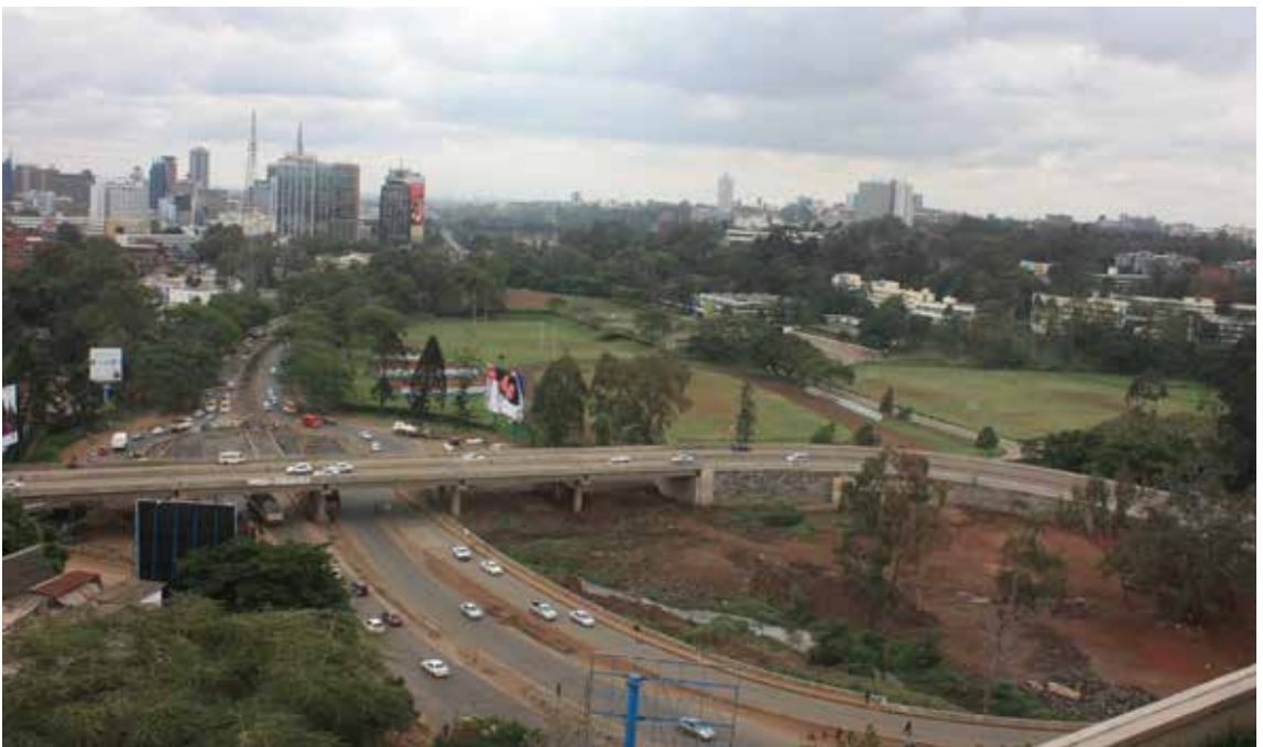
Construction of infrastructure in Nairobi, Kenya © Kenya Vision 2030
