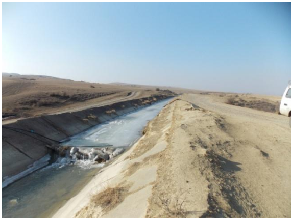
Raising water level by using material placed on the bottom of the canal
