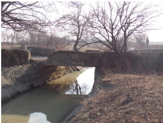
Drainage bridge over the canal
