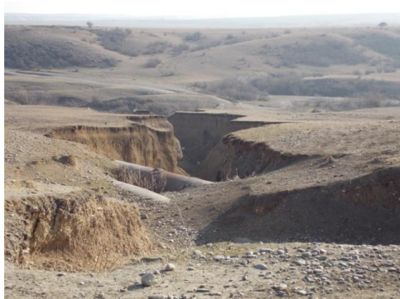
III inverted siphon corridor
