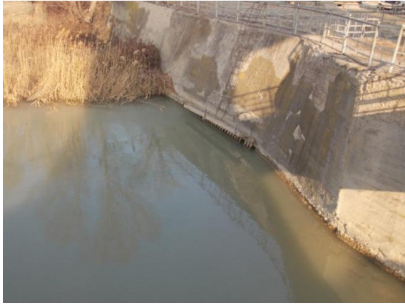
Inlet of water intake of the right main canal
