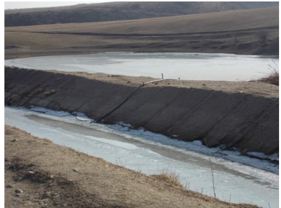
Unauthorized water abstraction and artificially arranged pond
