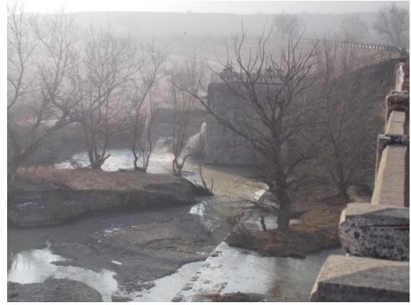
Tailrace, idle spillway
