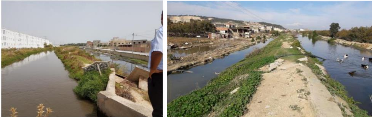
Picture A8.5 Low quality TWW conveyed through an open-air channel to the sea before the Project posing and environmental and health risks to the surrounding community. Source: ONAS
