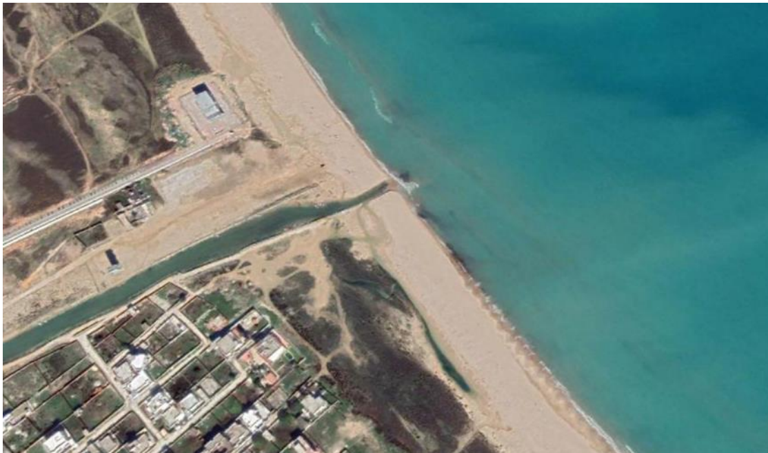
Picture A8.2 Clear sea water at Raoued beach and Khelij river after the construction of the submarine outfall. Source: ONAS
