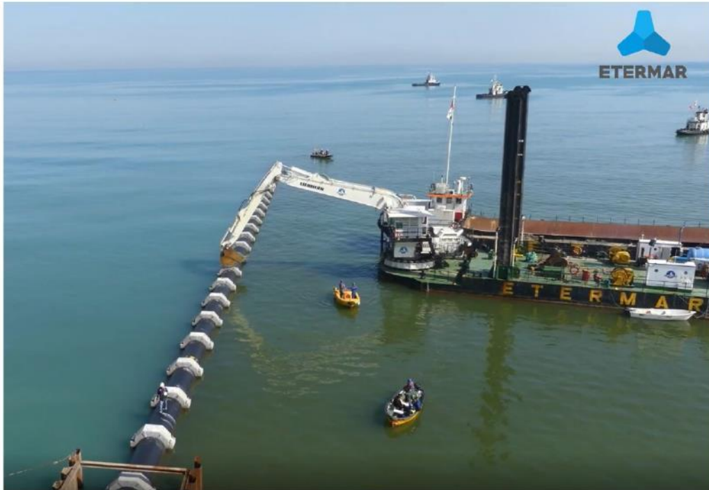
Picture A8. 3 Installation of submarine outfall. Source: ONAS
