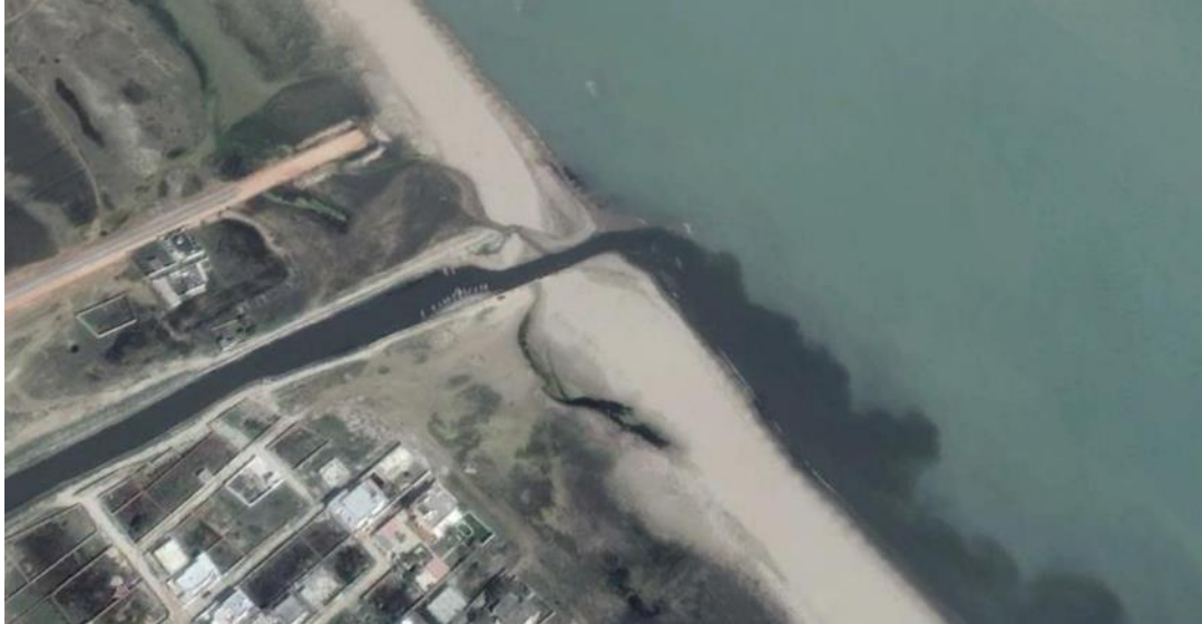
Picture A8.1 Contamination shown at discharge point of TWW at Raoued beach before the construction of the submarine outfall in 2015. Source: ONAS
