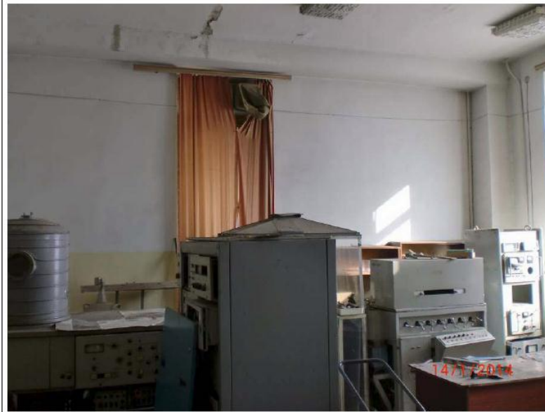
Main building 1. floor, Large laboratory room with flaking on the ceiling and beams (Force F)
