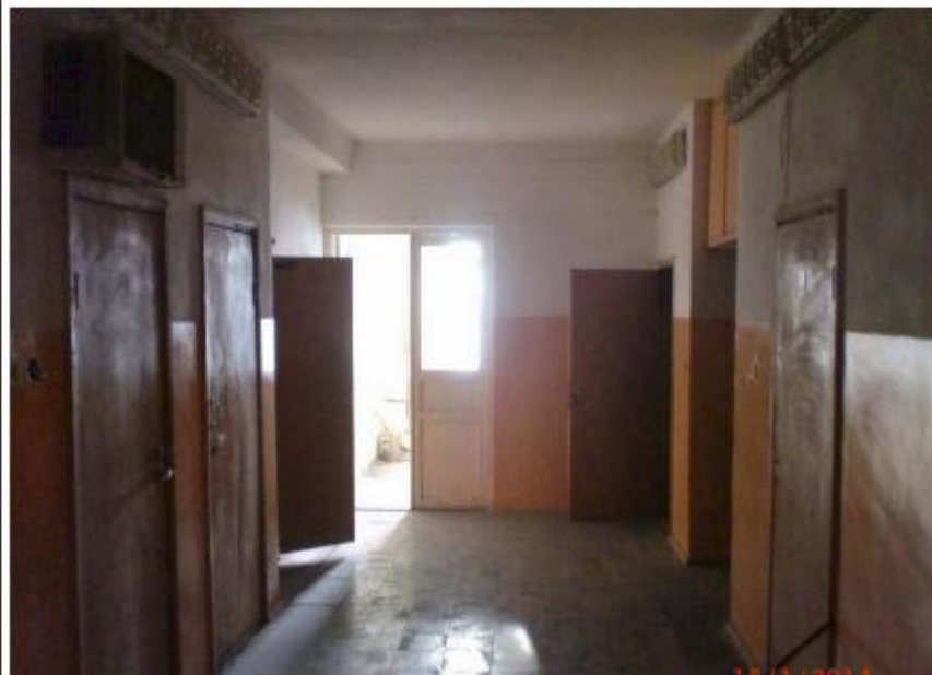
Main building 3. floor, Center aisle toward stairwell south side
