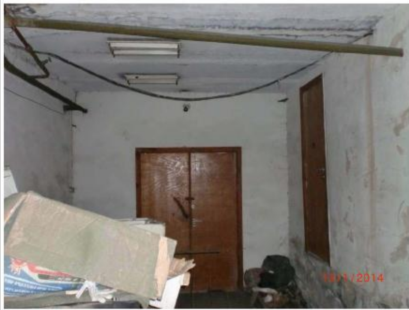
Main building basement, Side corridor (east side)
