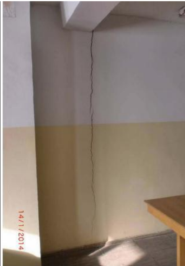
Main building 2. floor, Seminar room with tear-off wool to support (Dimensional L4)
