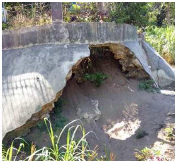
Figure 29. Intake Canal Wall at Jatimulyo, Dlingo, which was Damaged by Flood (left), and Riverbank at Tuk Pecah Magelang (right)
