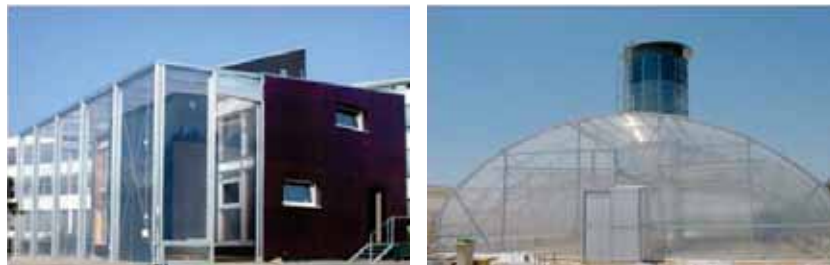
FIGURES 15 AND 16 The Watergy prototype in Berlin- Dahlem (Germany), South-Facing Greenhouse Facade; the Watergy Prototype in Almeria (Spain), Cooling Tower in its Center (right)
