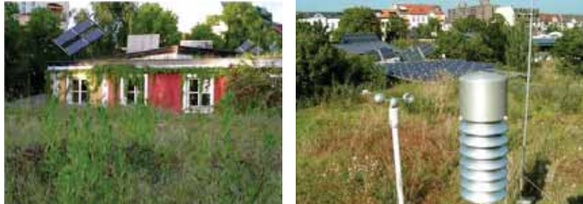
FIGURES 8 AND 9 Greened Roofs, UFA-Fabrik Berlin-Tempelhof (priority 2)
