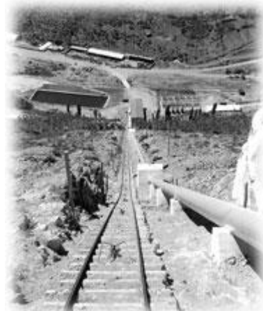
The funicular to Los Molles hydroelectric plant, 1953
