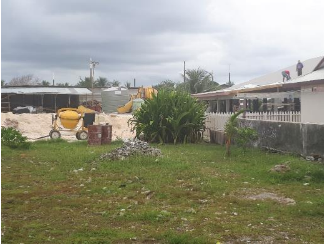
Figure 10: Nanumaga Island's community hall being built on the shoreline of proposed landing site 4
