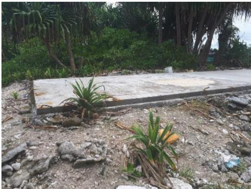
Figure 5: Concrete slab at vegetation line on proposed landing site 2
