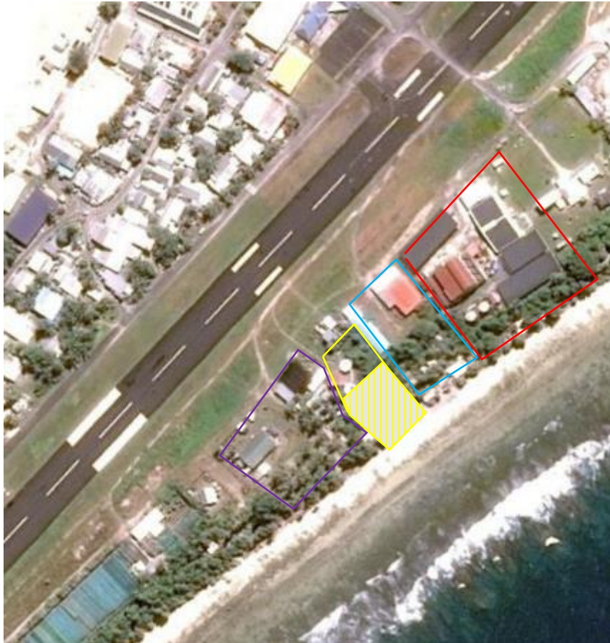
Figure 14: Potential Landing Site 5 (yellow) with the Tuvalu prison (purple), public meeting hall (orange) and Tuvalu Electrical Corporation (TEC) power plan and offices (red). Approximate extent of informal piggeries at site 5 in hatched yellow.
