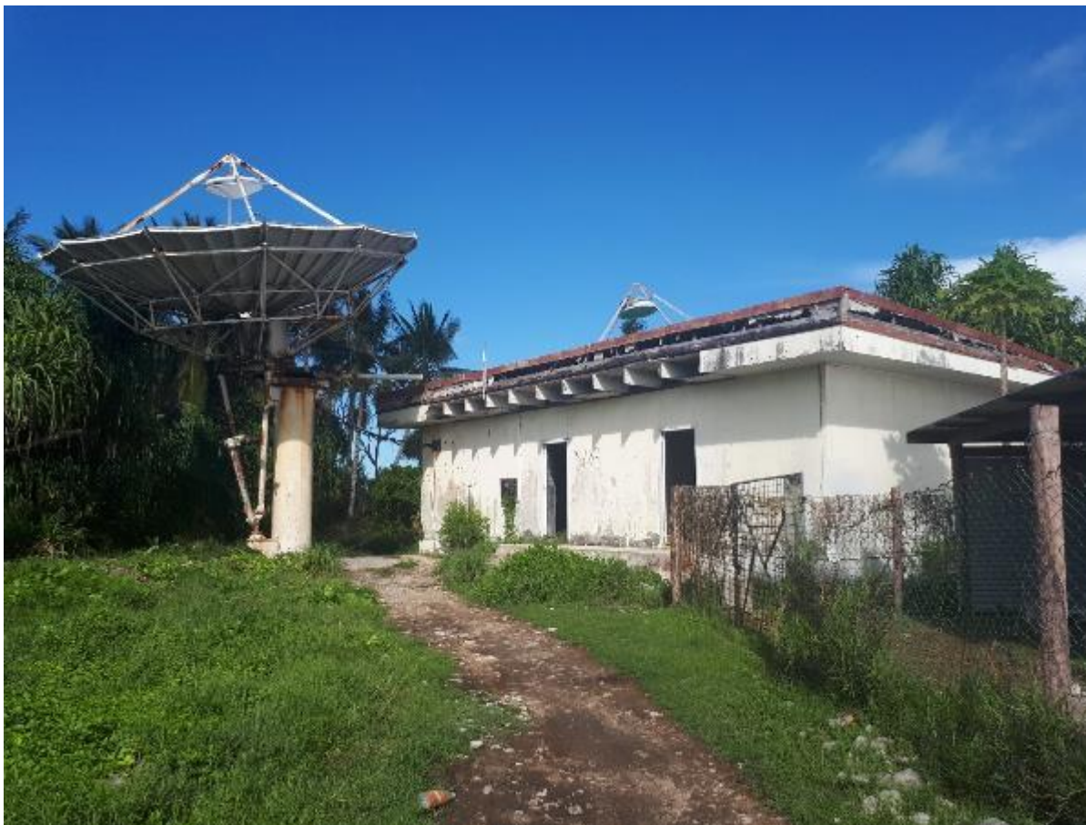
Figure 17: Disused building at proposed landing site 5
