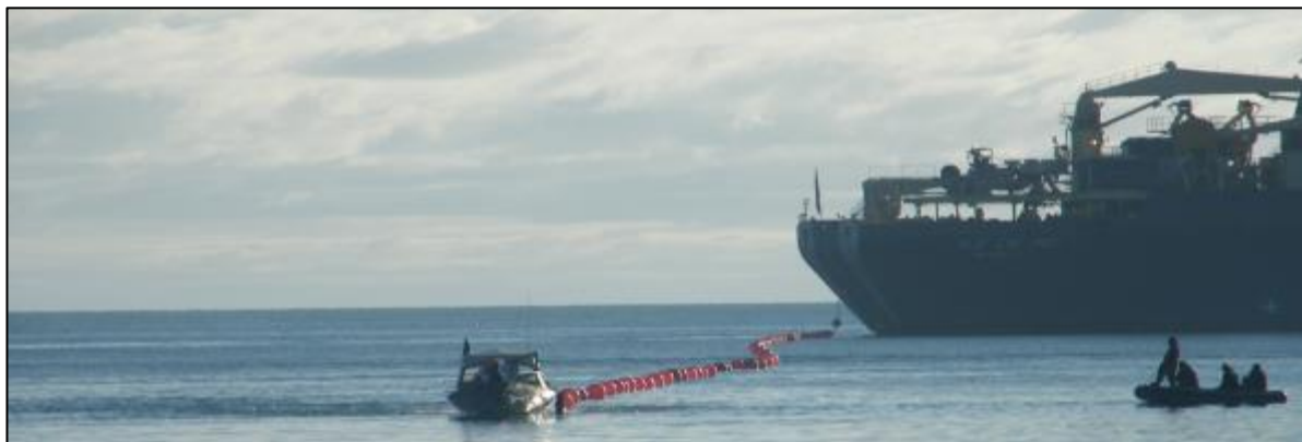
Figure 27: Cable landing operations, Nuku'alofa, Tonga
