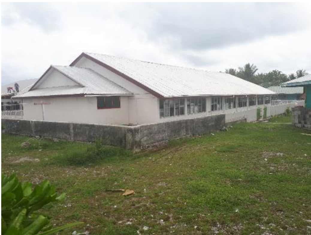
Figure 11: View of EKT church from the sea wall of propose landing site 4
