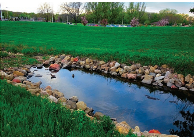
a. Stormwater retention pond
