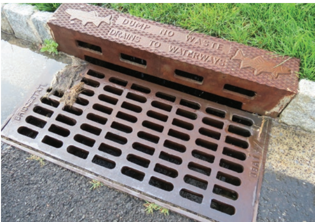
a. Catchpit grate
