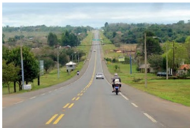
Rural road rehabilitation, Paraguay. Photo: World Bank
