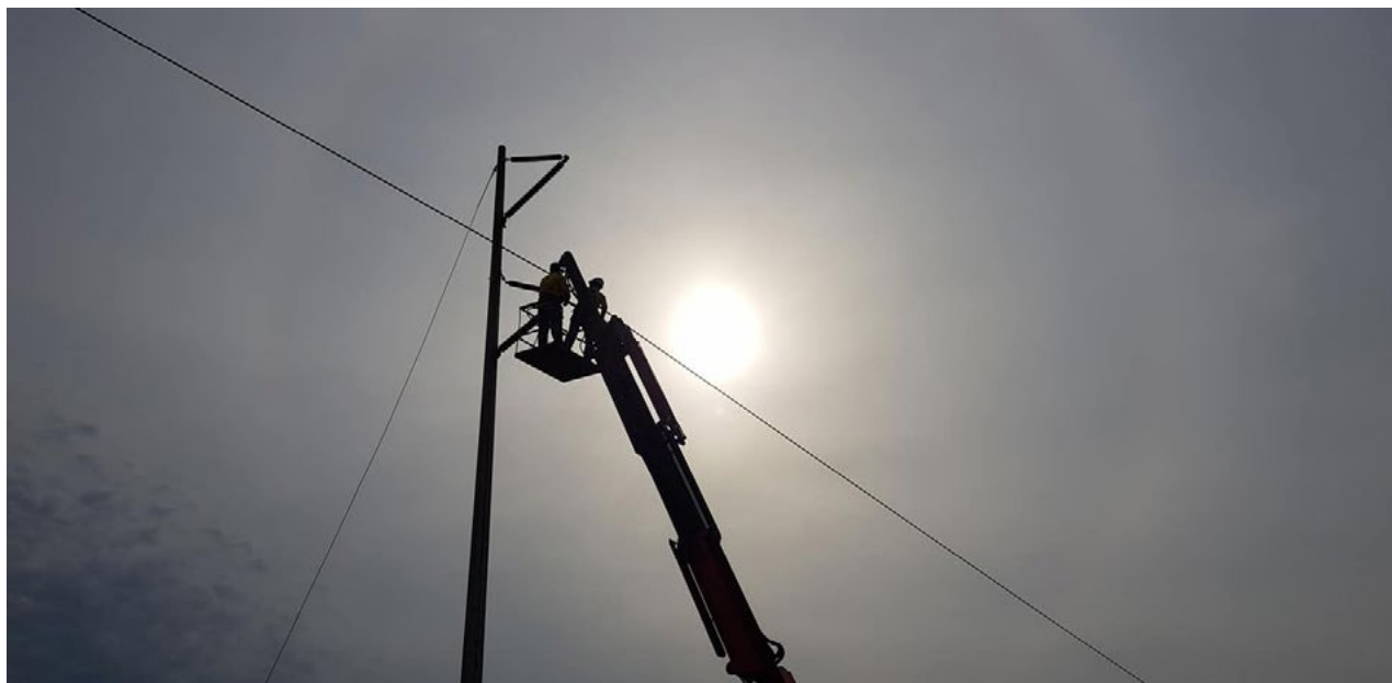
Power network maintenance, Paraguay. Photo: National Electricity Administration
