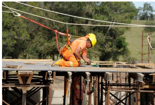
Sewage water plant construction, Uruguay. Photo: Presidencia Uruguay
