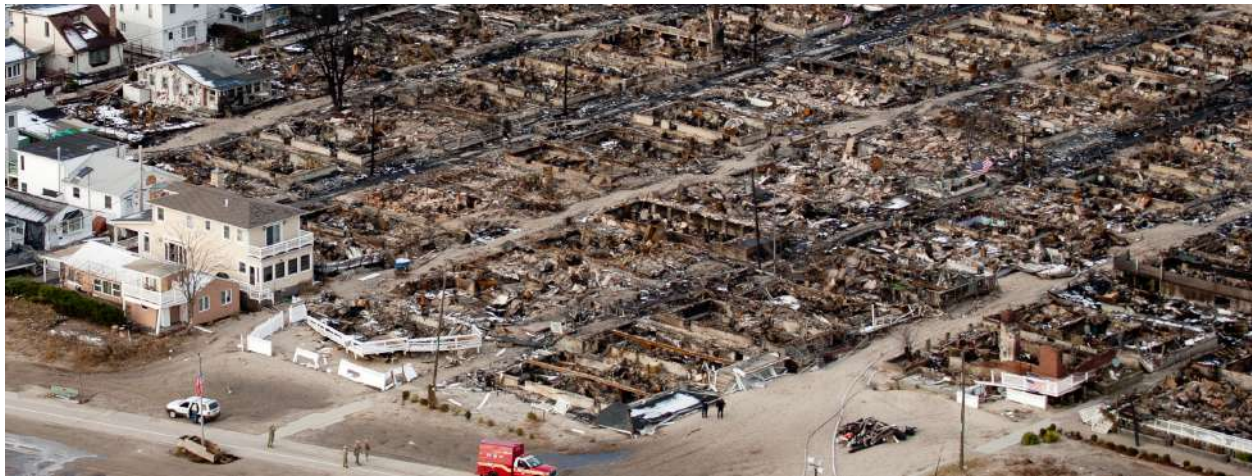
Figure 14: Aerial view of flood and fire damage caused by Hurricane Sandy, Breezy Point Neighborhood, Queens, NY, 2012
