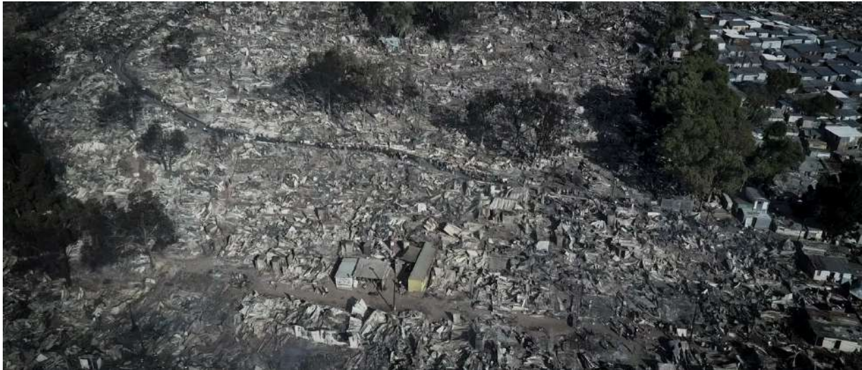
Figure 10: Aerial view of extent of damage following fire in an informal settlement, South Africa, 2018
