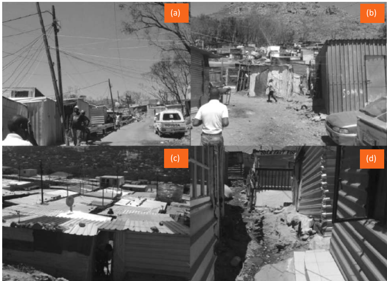
Figure 11: (a) Numerous illegal connections (all except top two lines) onto electrical infrastructure; (b) steep rocky terrain making access difficult; (c) dwellings located close to each other; and (d) narrow access ways between houses
