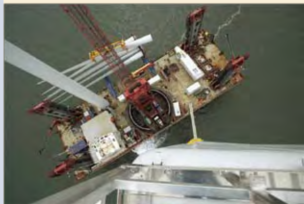
FIGURE B1.14: INSTALLATION OF WIND TURBINE AT BURBO BANK
