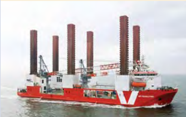
FIGURE B1.6: SPECIALIST WIND FARM INSTALLATION VESSEL: THE RESOLUTION
