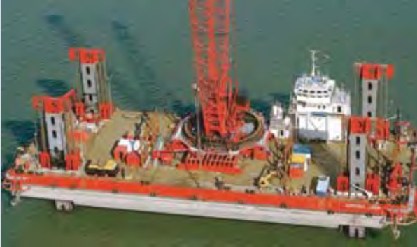
FIGURE B1.5: JACK-UP CRANE-BARGE: SEA JACK
