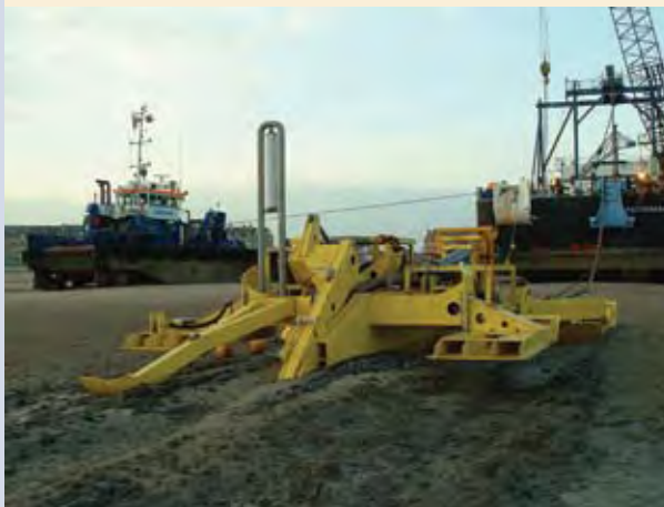
FIGURE B1.15: CABLE LAYING
