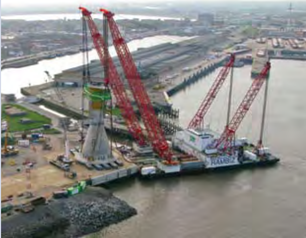
FIGURE B1.12: HEAVY LIFTING CRANE HANDLING GRAVITY BASE STRUCTURE
