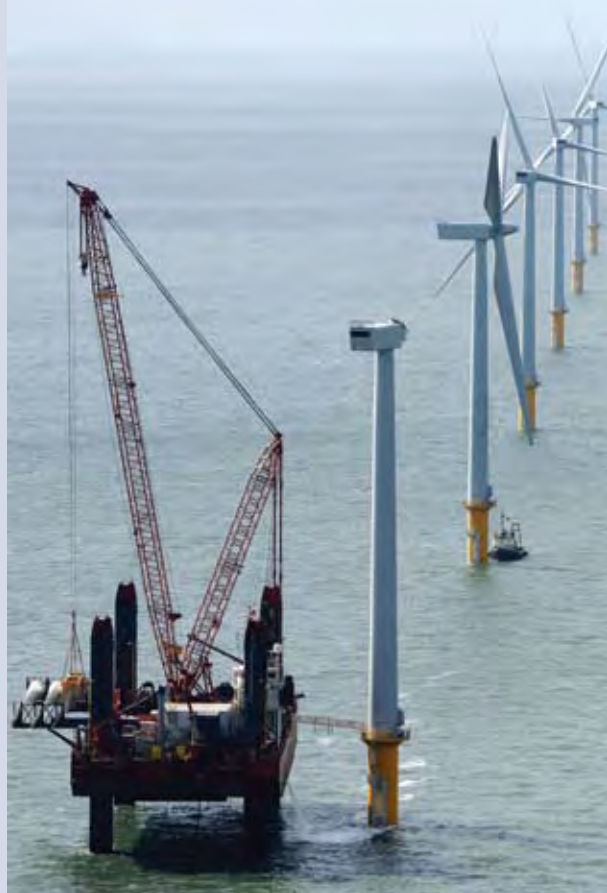
FIGURE B1.13: INSTALLATION OF WIND TURBINE AT BURBO BANK, UNITED KINGDOM
