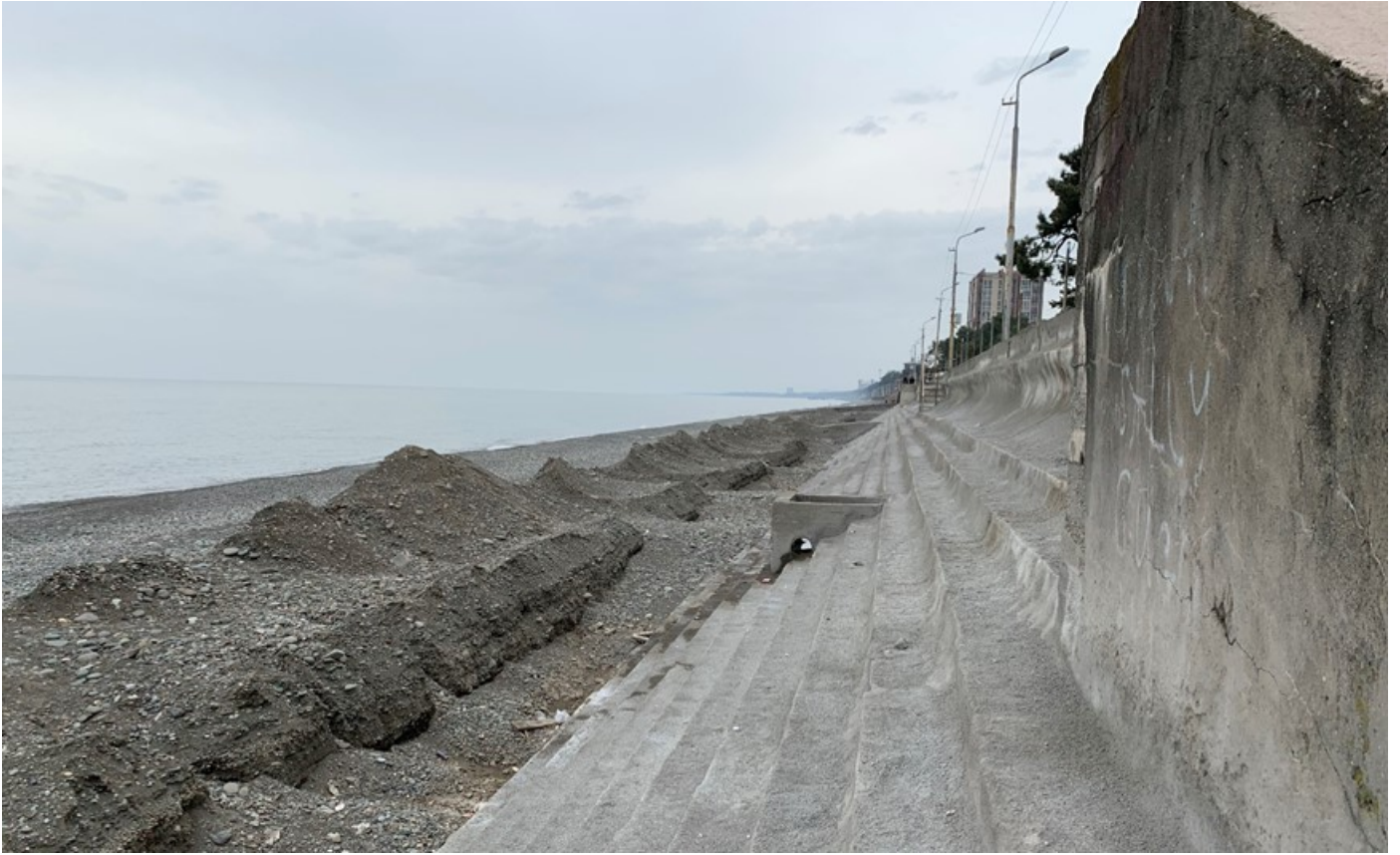
Coastline protection work north of Batumi Source: Sergio Vallesi. 2019
