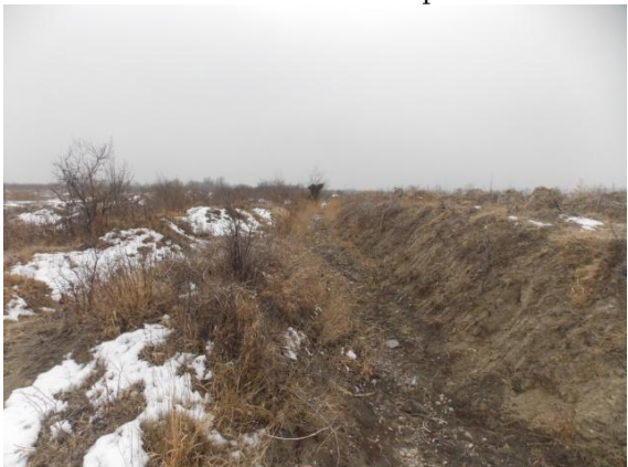
Main canal. pk104+00
