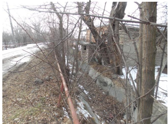
Main canal. pk154+20
