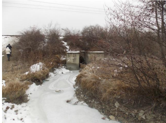
Crossing with the railway. pk72+00
