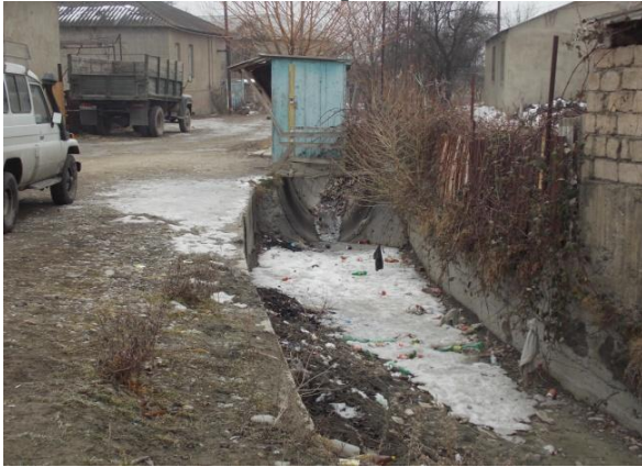
Main canal. pk122+00
