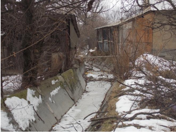
Main canal. pk120+00
