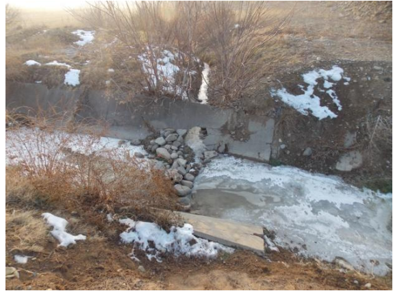
Main canal. pk257+00
