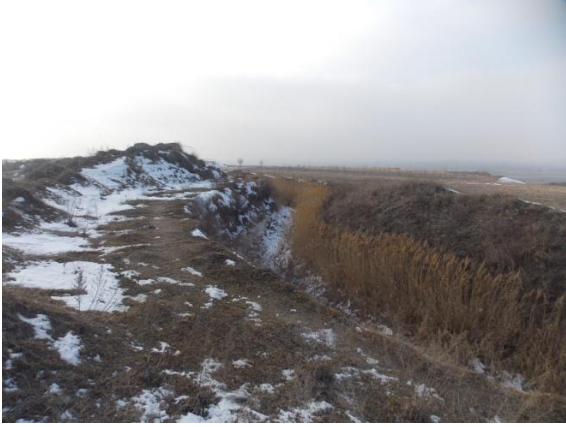
Main canal. pk176+00
