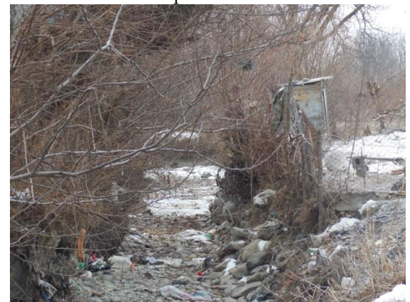
Toilet on the berm of the canal. pk37+30
