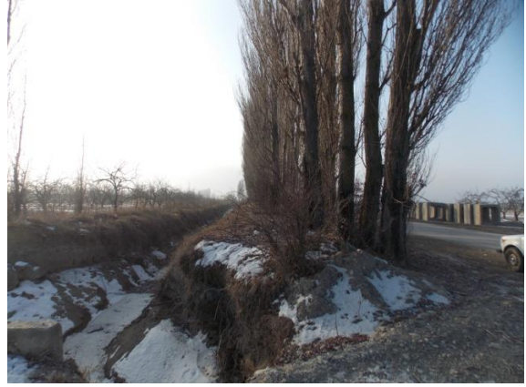
Main canal. From pk0+00
