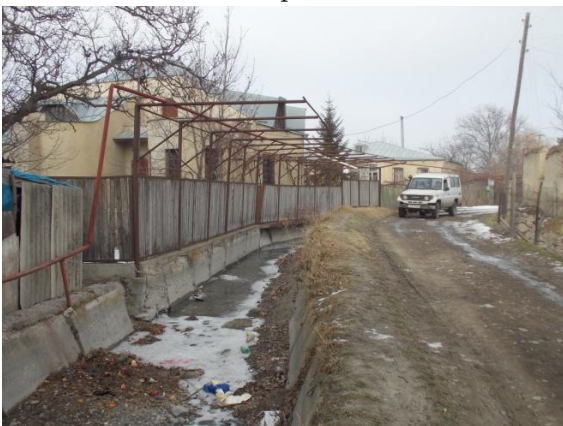
Main canal. pk153+40
