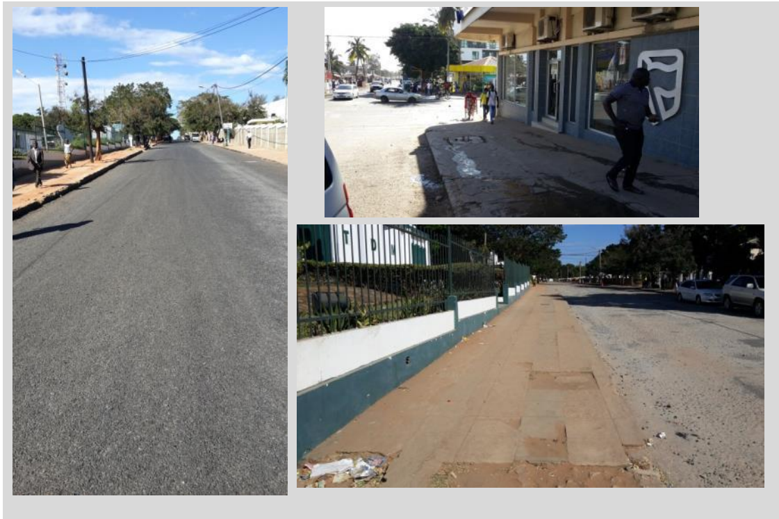
Figure 4-5: Paved areas and roads potentially to be degraded for pipes exchange in Pemba
