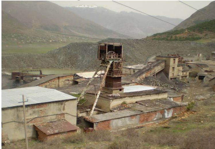
Picture 1: Bulqiza chromite mine, entrance
