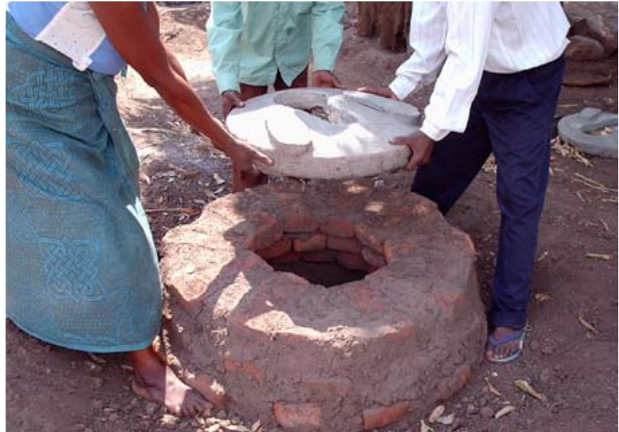
Installing small slab on bring ring beam for Arborloo Photo Credit: Peter Morgan
