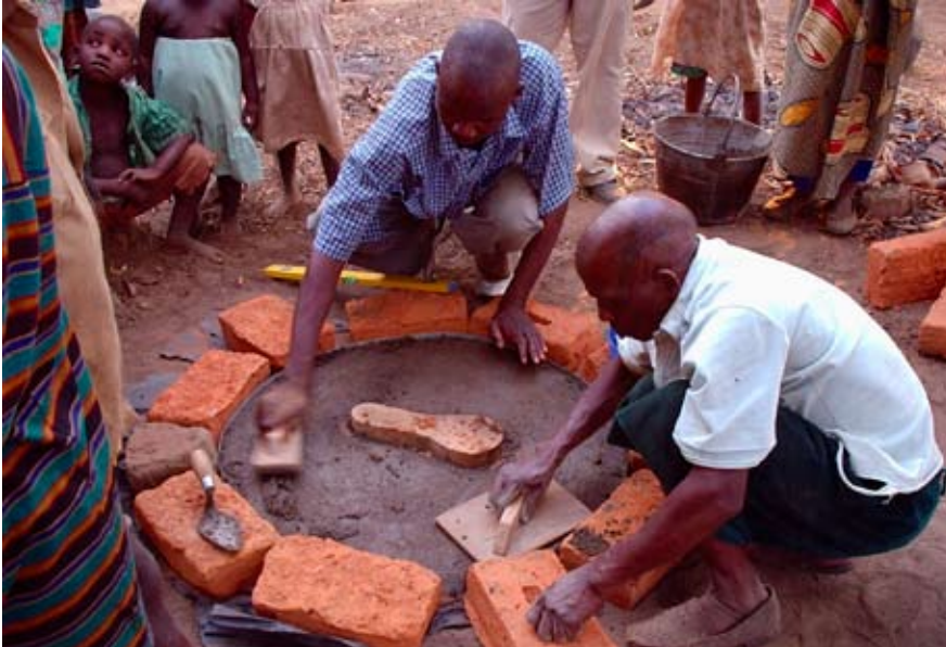
Making concrete slab for eco-toilets, Malawi Photo Credit: Peter Morgan
