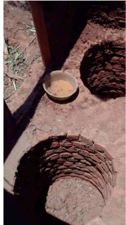
Twin pits in a Fossa alterna, Thyolo. Photo Credit: Peter Morgan
