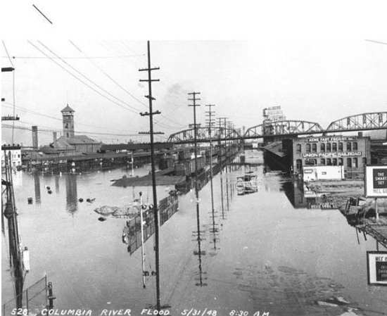
Figure 12: Flooding in Portland, OR (Source: USACE, Portland District, photo archive)
