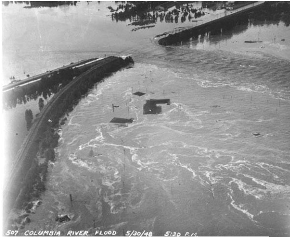
Figure 11: Flooding in Vanport, OR (Source: USACE, Portland District, photo archive)
