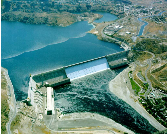
Figure 13: Grand Coulee Dam (Source: US Bureau of Reclamation, photo archive)
