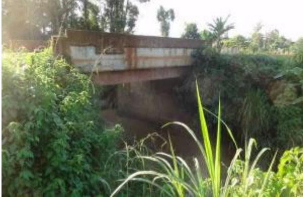
Photo 6-17: Km 52.30 Namatala Bridge deck
