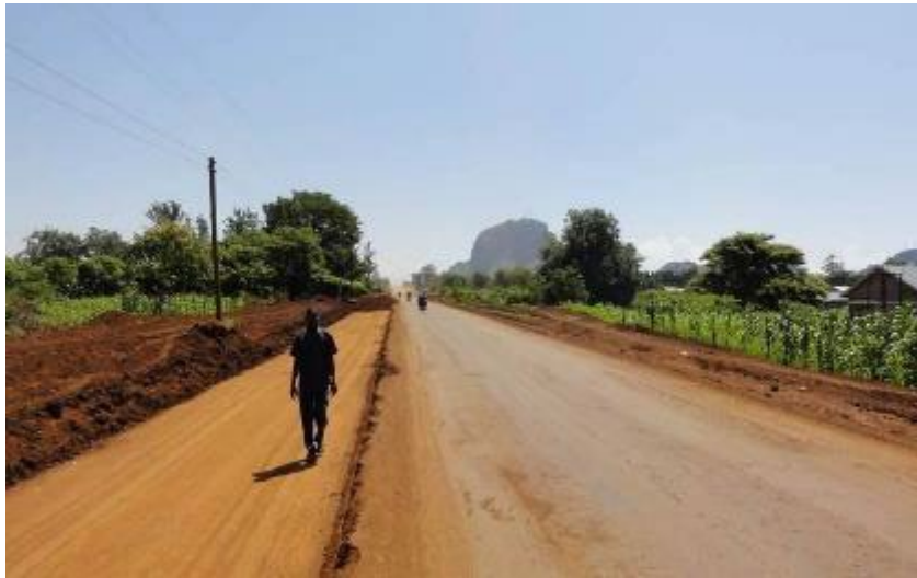
Photo 1-4: Lot 1, Km 0.5, May 2013, Widening by benching south of Tororo
