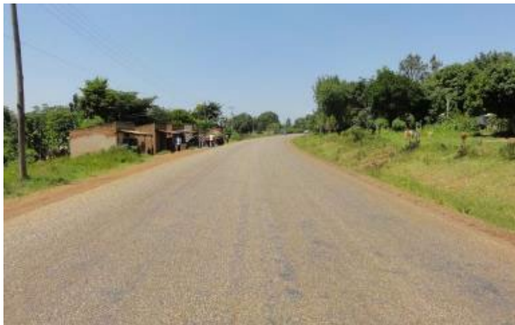
Photo 1-15: Horizontal Curve at km 31 on southern approach to Manafwa Bridge
