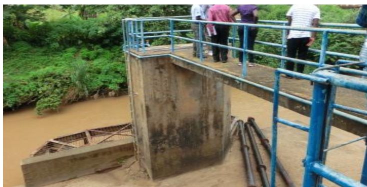
Photo 6-12: Km 31.77 Manafwa Bridge, composite deck, edge beam and railings
