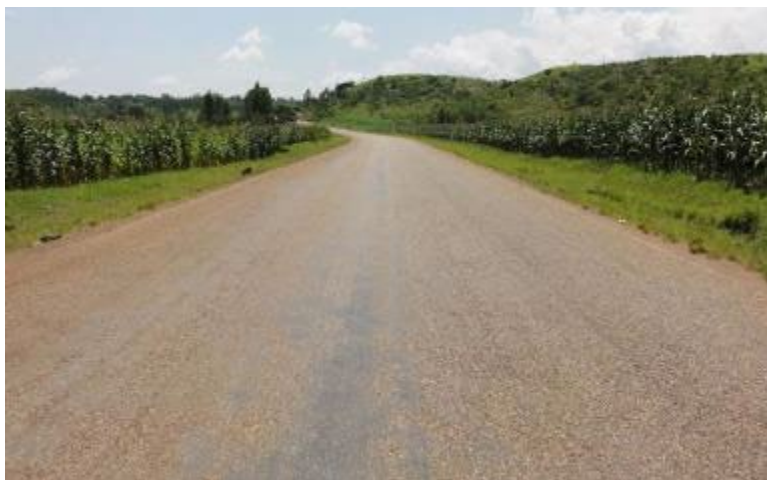
Photo 1-16: Horizontal Curve at km 32 on northern approach to Manafwa Bridge
