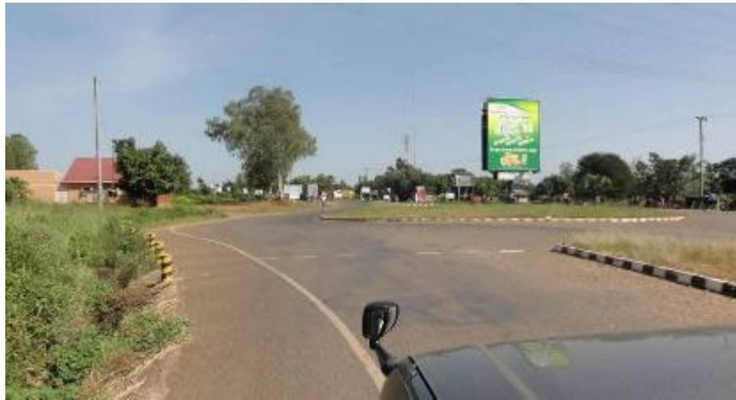
Photo 1-10: End of Lot 2 / Start of Lot 3 at end of Lira Bypass
