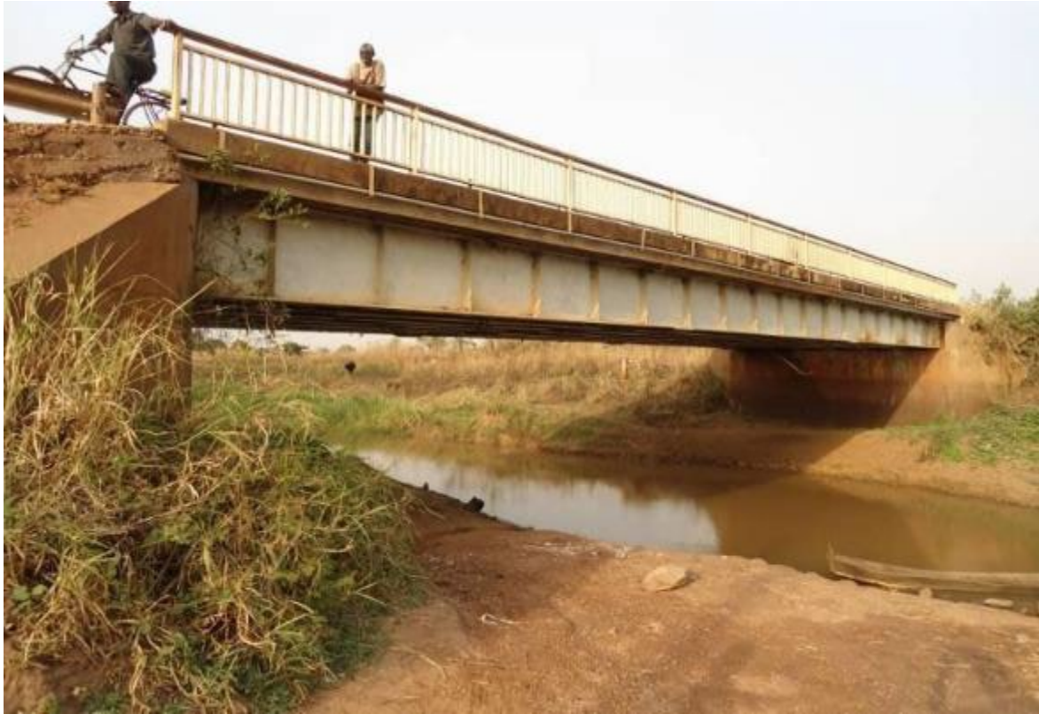
Photo 6-23: Tochi River Bridge on Lira-Kamdini Section Km 63-65
