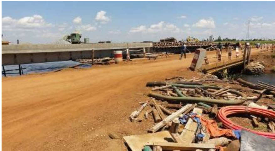
Photo 1-7: Lot 1, Km 134, New Awoja Bridge under construction
