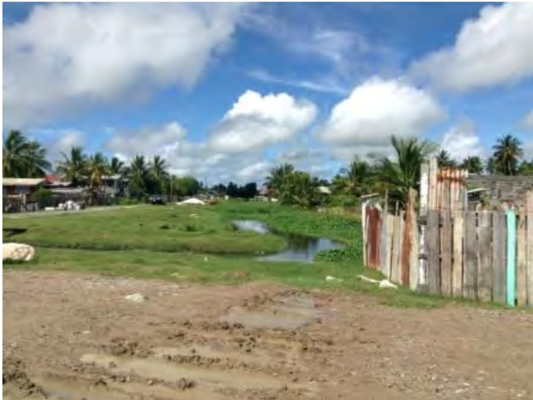
Figure 4.1: Access Dams in State of Disrepair (Buxton)
