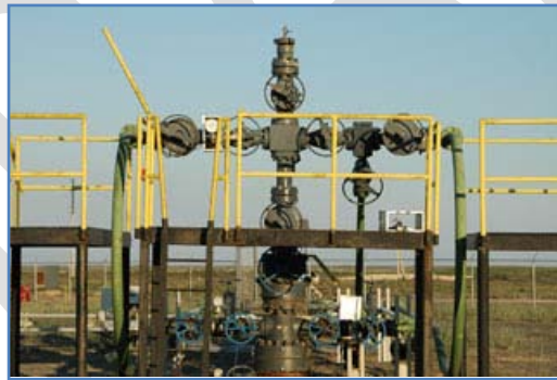
Figure 20: Oil well wellhead. [16]
