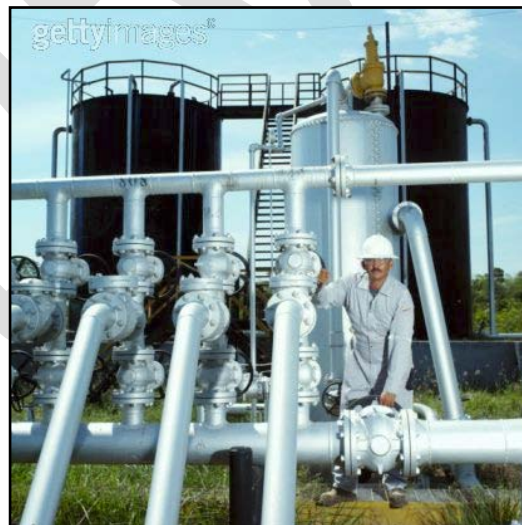
Figure 15: Header at a gathering station [14]
