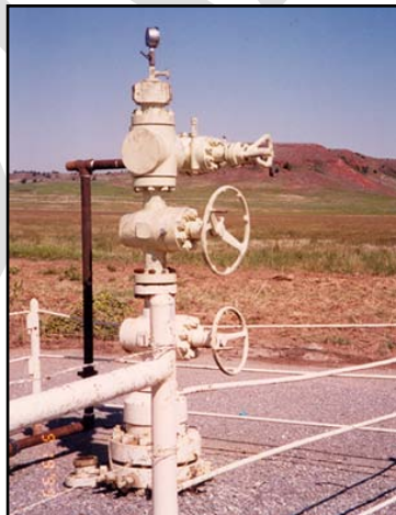
Figure 13: Typical gas well wellhead [13]
