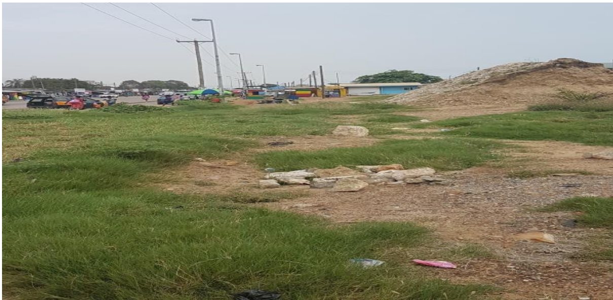
Section of Naval base site for the proposed drains construction
