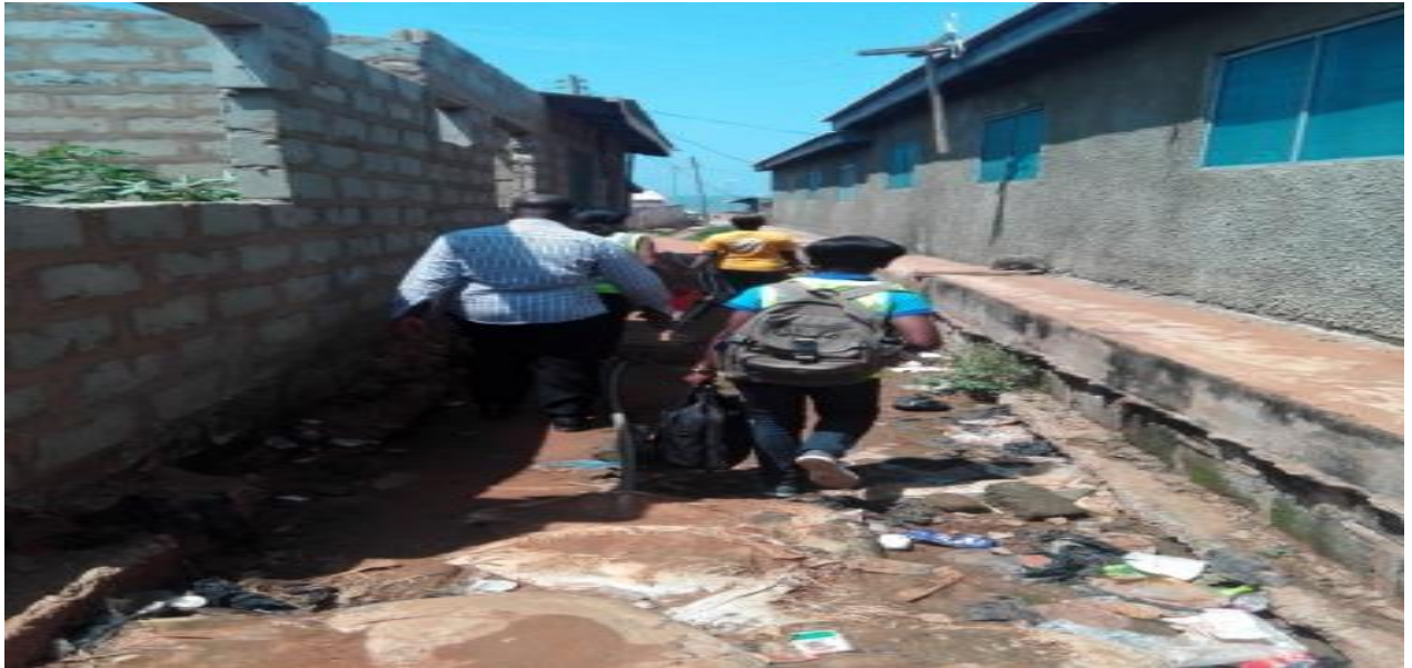
Earth drain course in Bankuman where drains will be constructed and slapped
