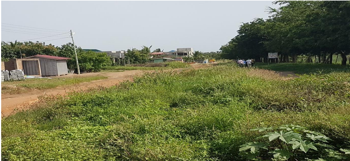
Adjei Kojo/Kanewu - An existing street corridor providing runoff direction where drains will be constructed to channel storm water away from the community
