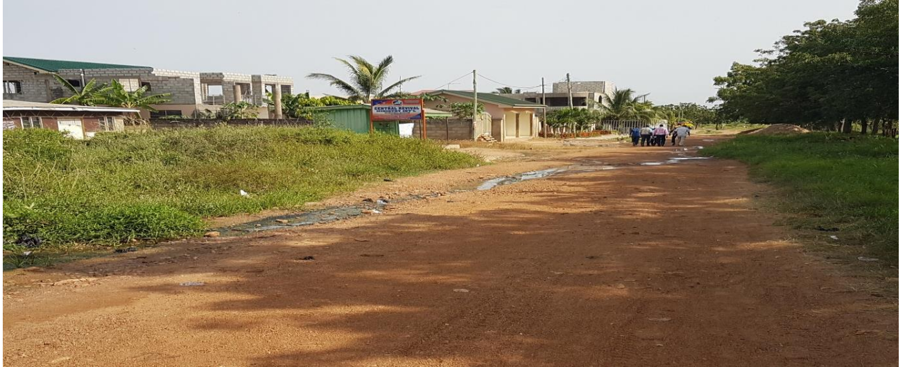
Adjei Kojo/Kanewu - An existing street corridor providing runoff direction where drains will be constructed to channel storm water to leave the community
