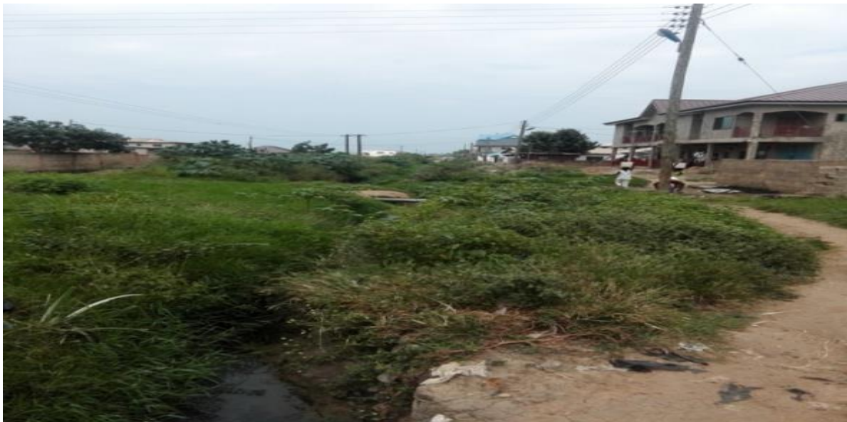
Adjei Kojo/Kanewu- A proposed drainage course under the project
