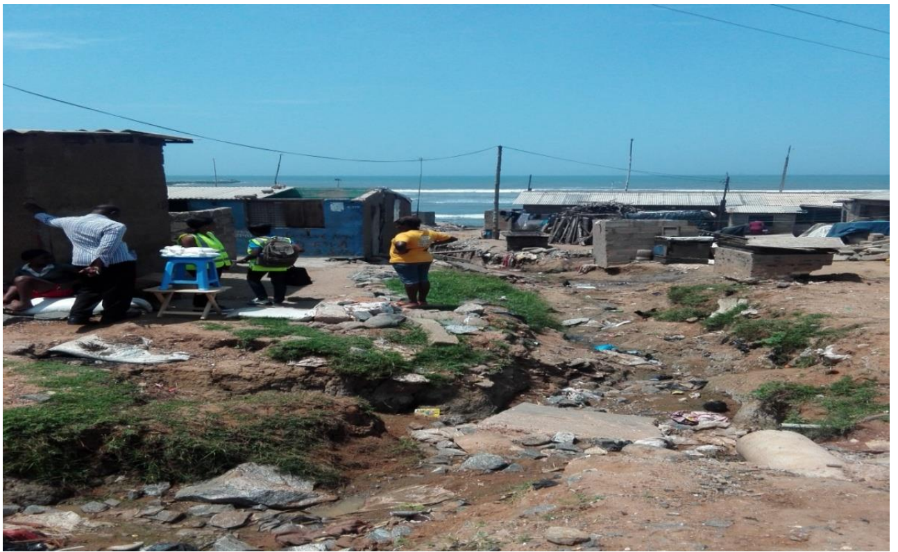
Earth drain route where drain will be constructed and slapped in Bankuman community
