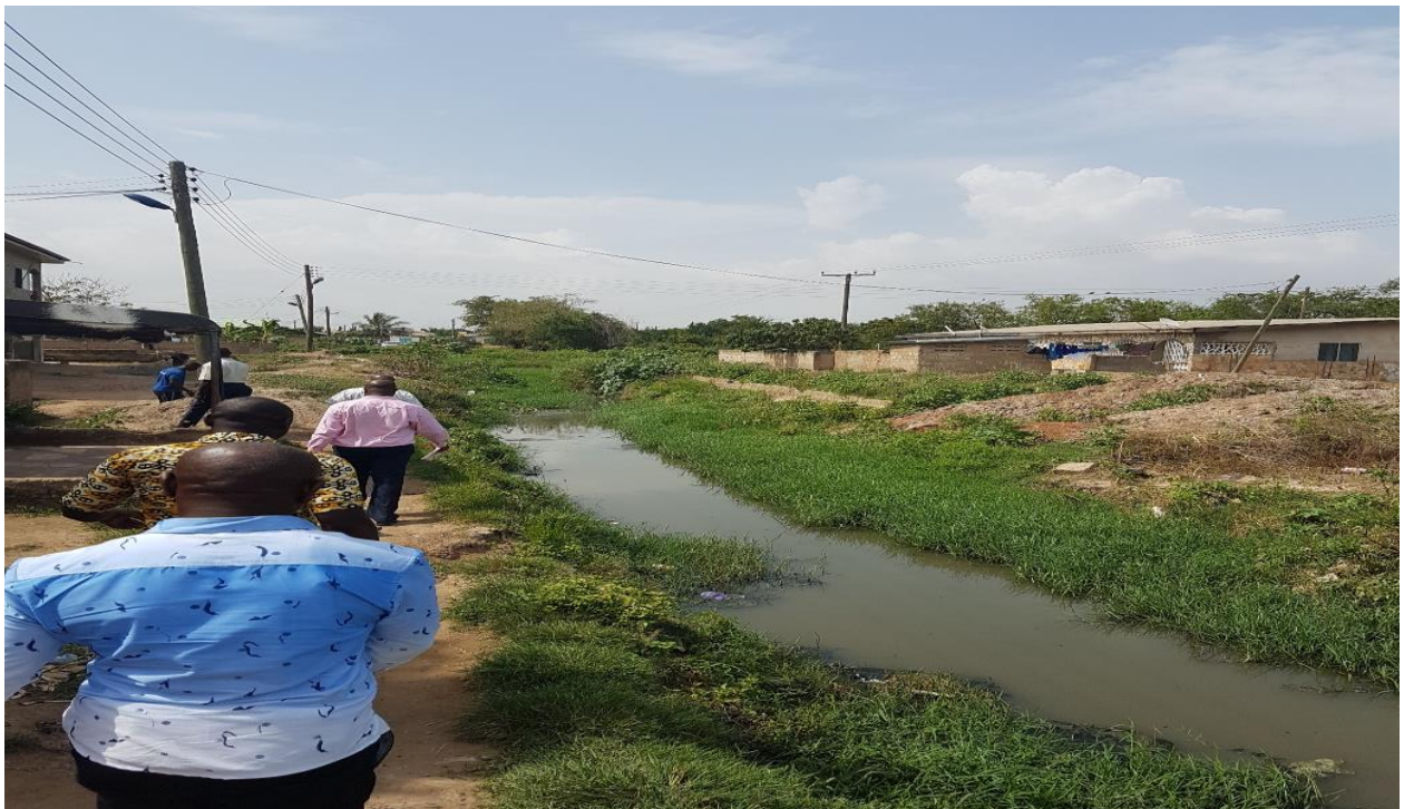
Adjei Kojo/Kanewu - An existing street corridor providing runoff direction where drains will be constructed to channel storm water to leave the community
