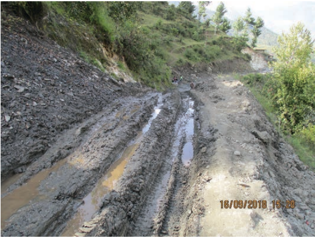
PHOTO 6.4 Road surface damage caused by seep created by a road opening, Mugu, Nepal
