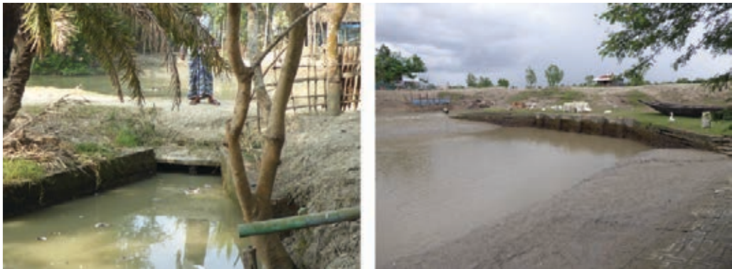
PHOTO 5.8 Use of turfing combined with jute netting
