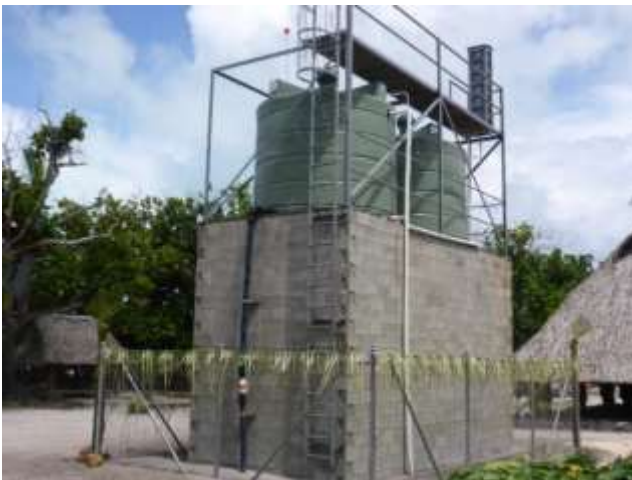
(Left) Storage head tanks at Notoue village in North Tarawa—part of the Notoue groundwater abstraction system. (Right) Replacement babai (taro) pit adjacent to the Notoue groundwater gallery reserve area.
