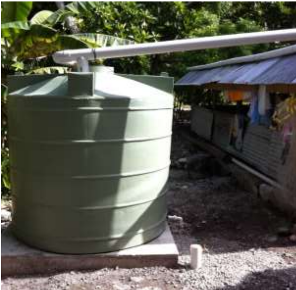
Rainwater harvesting tank, guttering, and connection pipes installed at a site in Makin Island under the Resilience Fund activities. Left: village building; right: community church.
