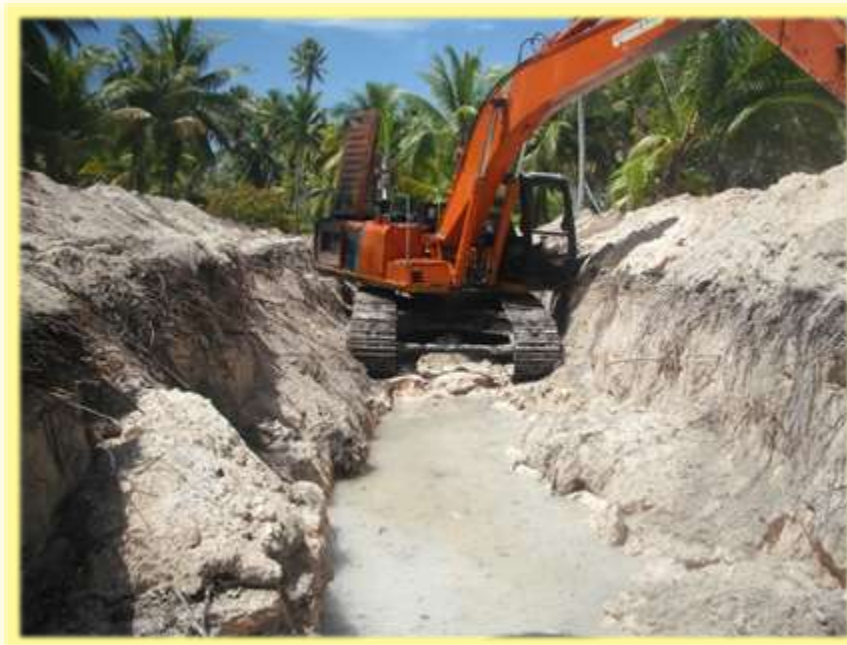
Excavation of groundwater abstraction gallery.
