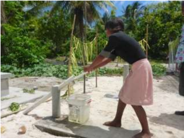
Tamana pump being operated. This is representative of several Tamana pumps installed in the Outer Islands.
