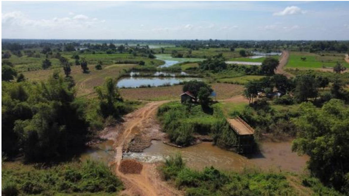
Existing bridge (right) and existing temporary detour (left)
