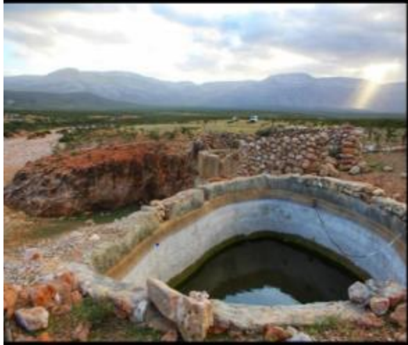
Rainwater harvesting reservoir 150 m 3 capacity – Tara'a - Qulansiyah and Abdulkoury – Socotra Governorate
