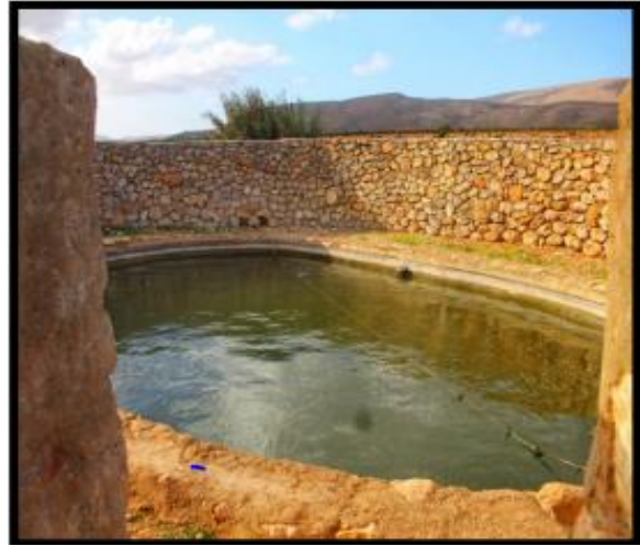
Rainwater harvesting reservoir 150 m 3 capacity – Tara'a - Qulansiyah and Abdulkoury – Socotra Governorate
