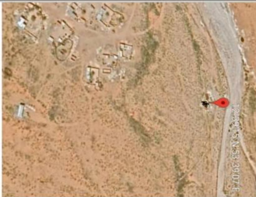
Rainwater harvesting reservoir 85 m 3 capacity – Abtari – Moghabhar -Nujd – Hadibu Socotra Governorate
