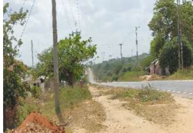
Pipeline route free from encroachment
