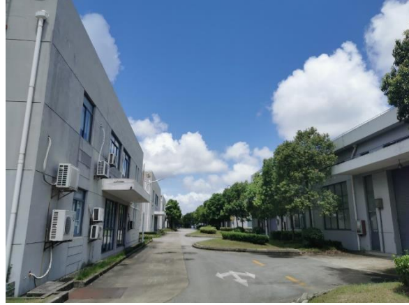
Photo 14: Eastern boundary of the No.3 building.
