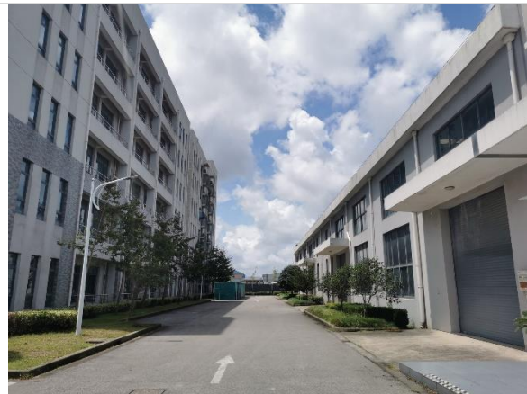
Photo 15: Southern boundary of the No.3 building.
