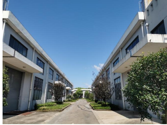
Photo 13: Northern boundary of the No.3 building.
