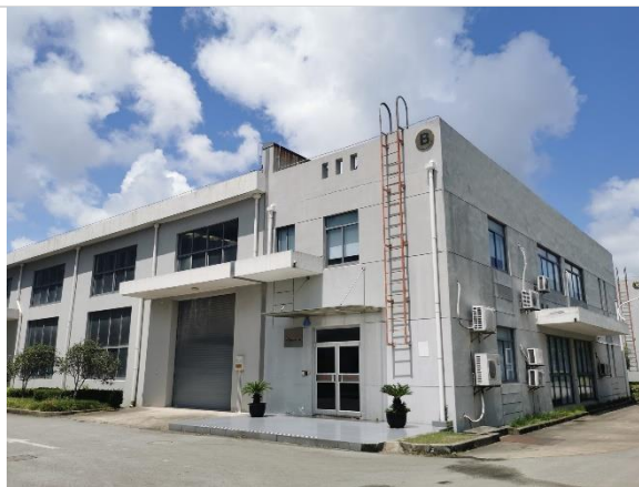
Photo 2: Entrance of WFS (No.3 building)
