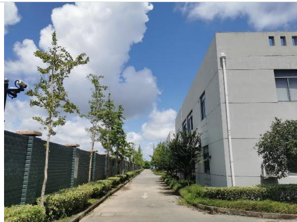
Photo 16: Western boundary of the No.3 building.
