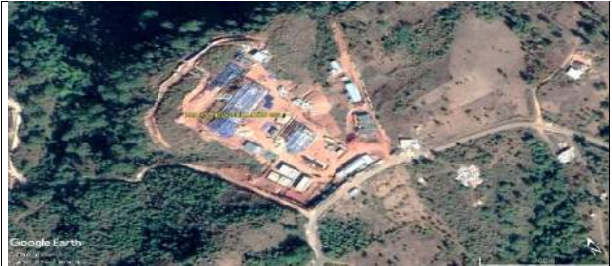
220/132 kV New Shillong
