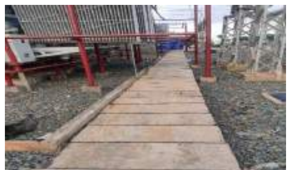
Plate 5.6 : Drainage constructed inside 220/132kV New Shillong
