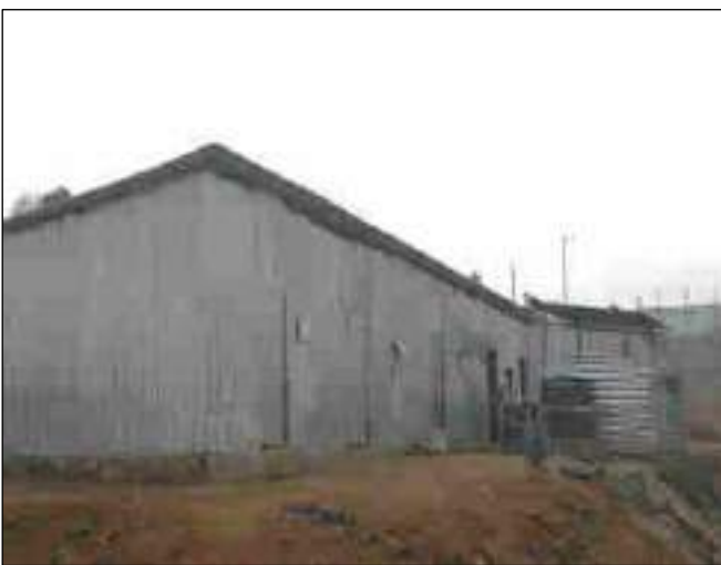
Labour camp at 220 kV New Shillong SS
