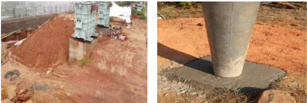
Plate 5.8: Backfilling & resurfacing of excavated area inside substation and 33kV pole
