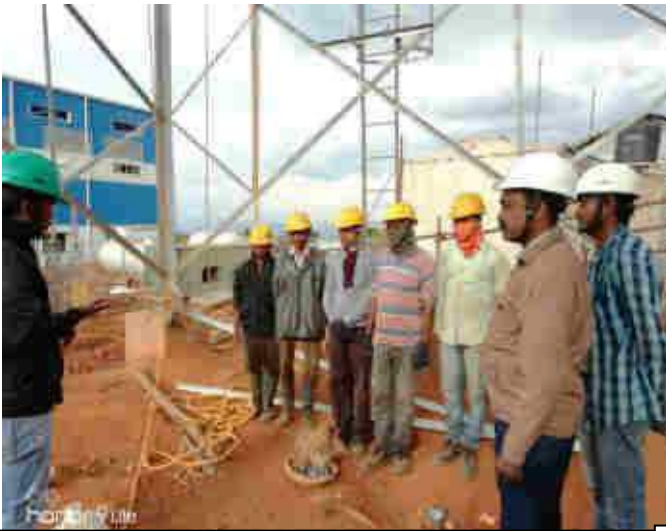
Height work training at Mawngap GIS Substation
