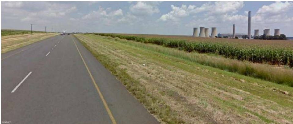
Figure 90: South-western view along R35 (KPS visible on right-hand side) (Google Earth™)
