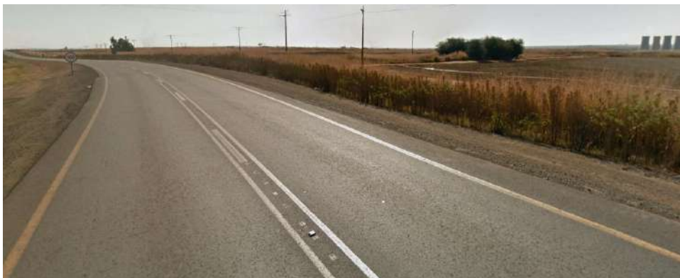
Figure 91: Western view along R35 (KPS' western cooling towers visible on right-hand side) (Google Earth™)
