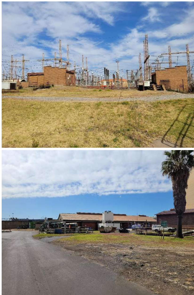
Figure 70: Photographs of grassed areas next to HV Yard (top) and eastern cooling towers (bottom)
