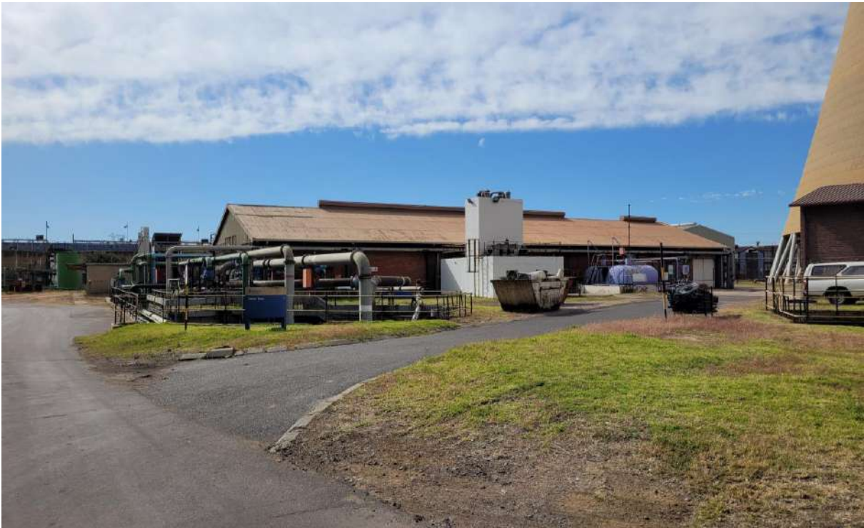
Figure 77: View of water treatment plant at KPS
