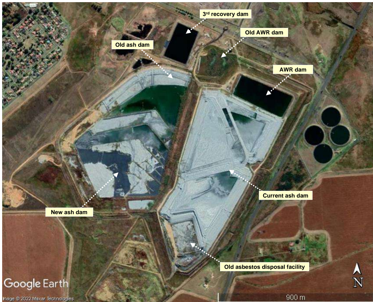
Figure 10: KPS ash dam area (Google Earth™)
