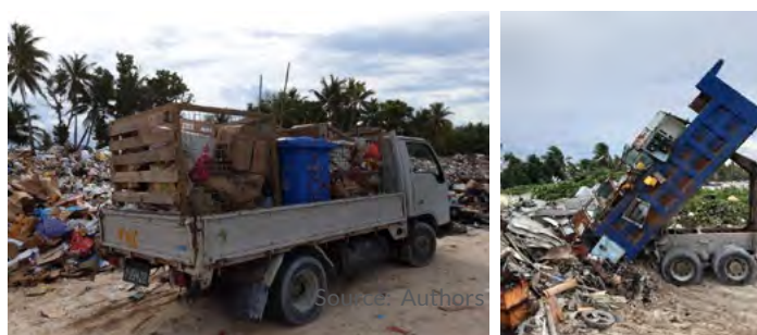
Figure 20: Hauling Waste. Commercial premises self-hauling waste and a mixed construction load.
