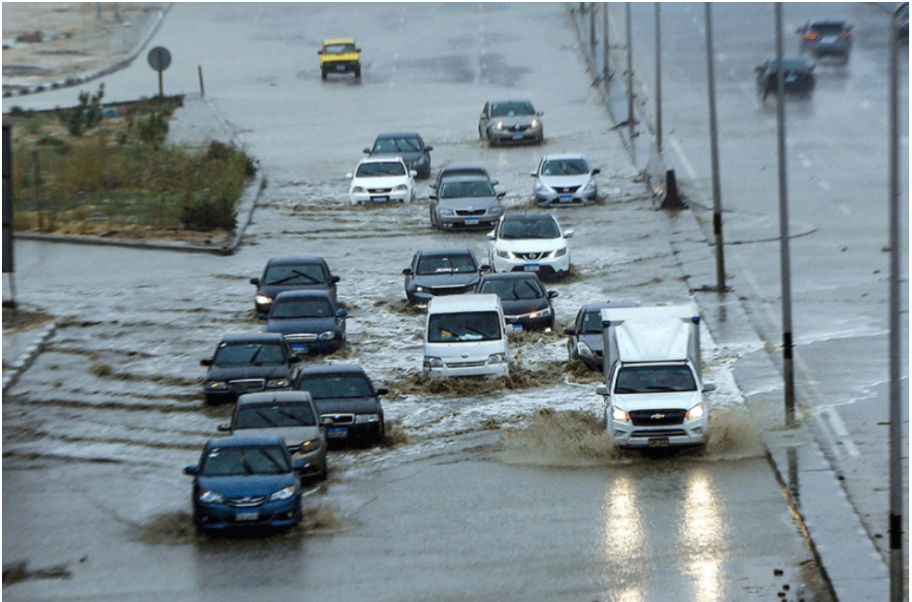
Flooding on roads in Qena, Egypt. © AFP
