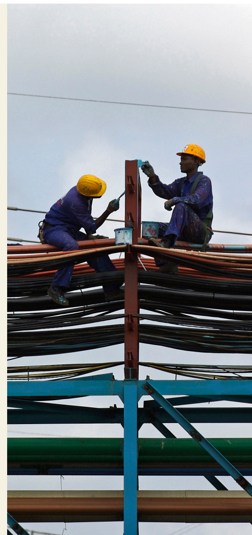
Workers maintain thermal power station in Ghana © Jonathan Ernst / World Bank
