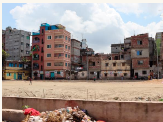
Example of neighborhood buildings and open spaces in Dhaka city. Photo from TDLC FY20 Annual Report.
