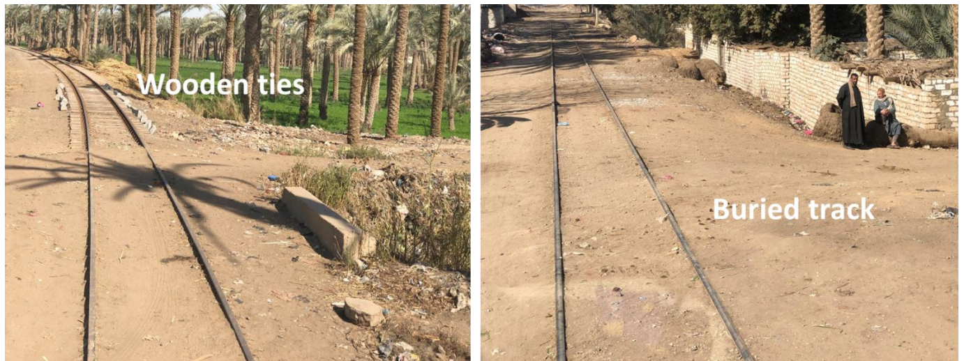
Figure 4-41: Segment 2 wooden ties and buried track
