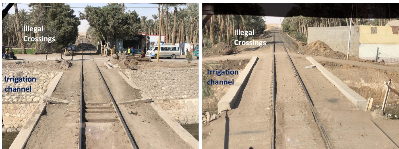
Figure 4-43: Illegal crossings and overpasses crossing small irrigation channels and local roads
