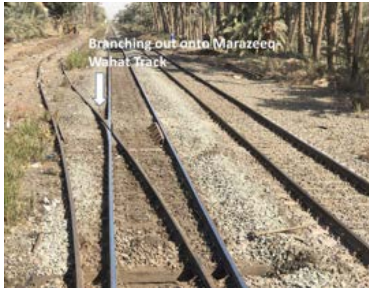
Figure 4-40: Branching out onto Marazeeq-Wahat track, i.e., segment 2
