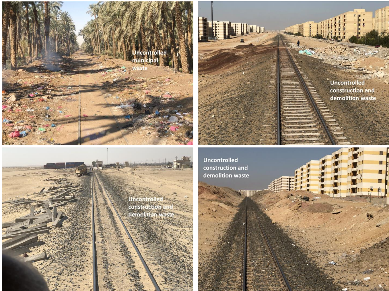
Figure 4-54: Uncontrolled disposal of waste along segment 2
