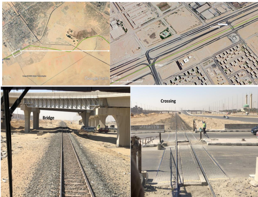
Figure 4-52: Segment 2 crossing local road off Wahat highway and going under bridge
