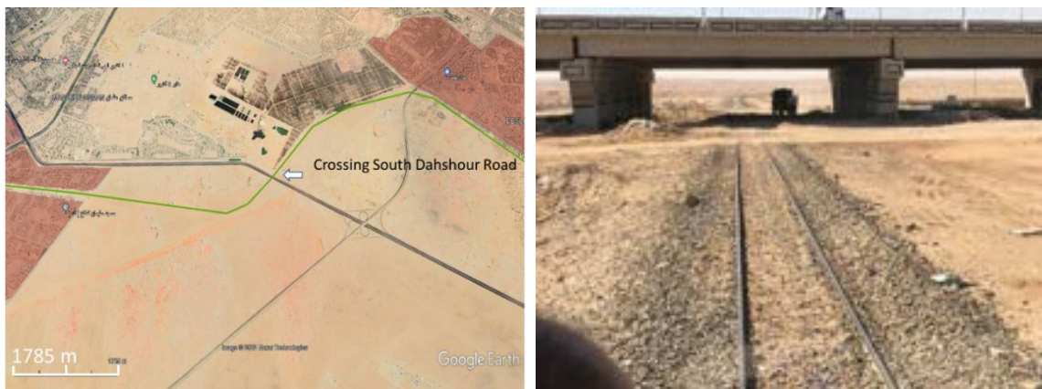
Figure 4-50: Segment 2 crossing under South Dahshour bridge
