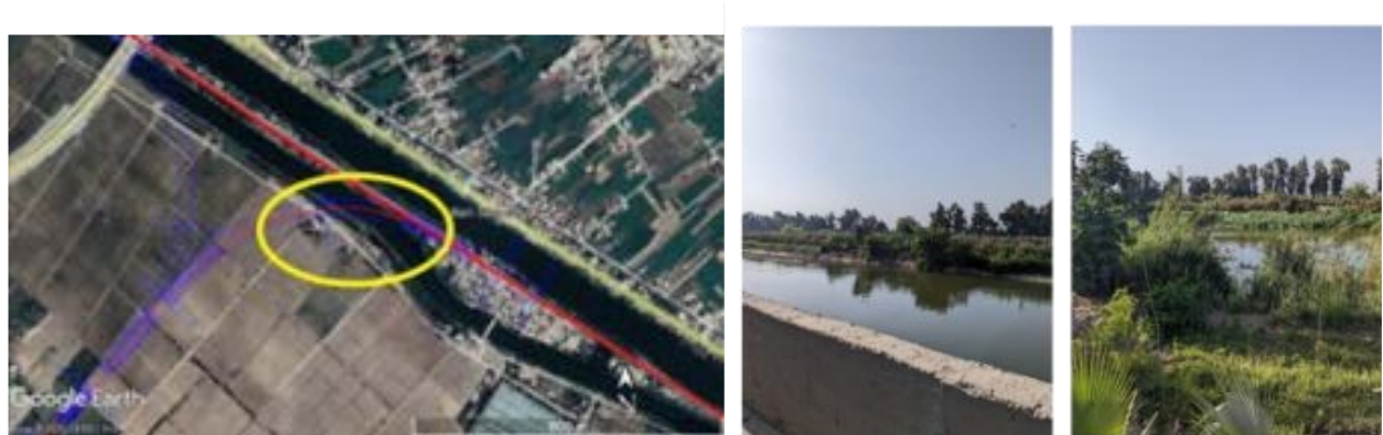
Figure 4-28: Reyah El Nassiri Channel crossing to link Itay Al Baroud-Bashtel line to the Bani Salamah-6th of October line
