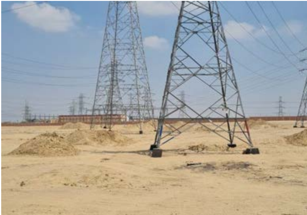
Figure 4-12: Power station near 50.5 KM in segment 1
