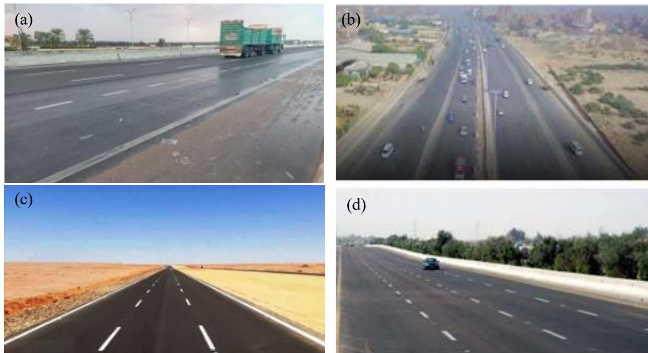
Figure 4-14: roads relevant to Segment 1: (a) El Wahat Road, (b) Regional ring road (c) Al Dabaa corridor, (d) Cairo-Alexandria desert road
