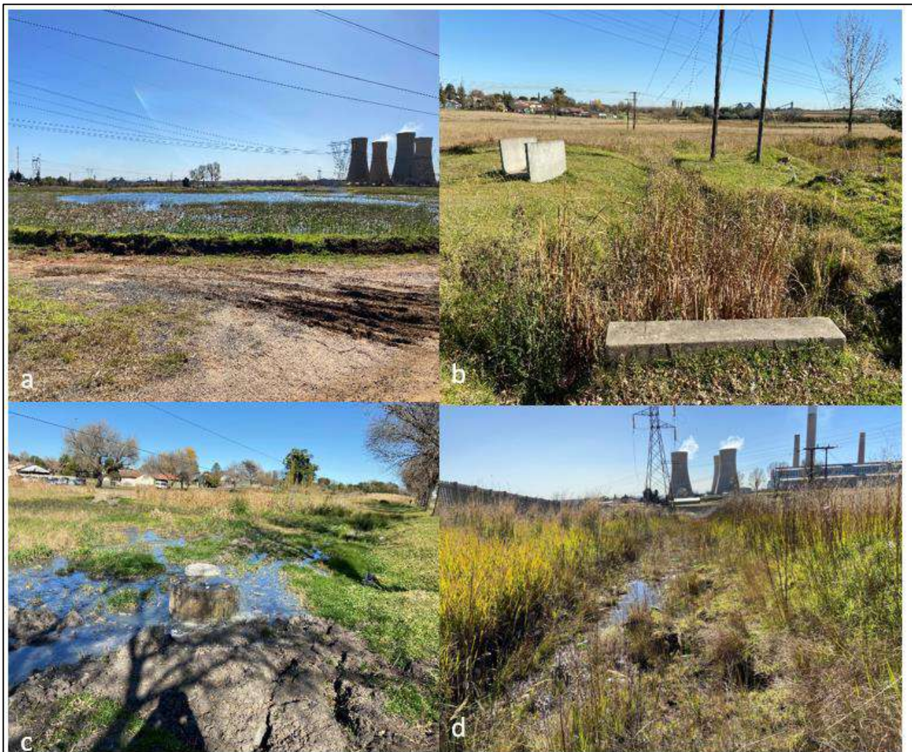
Figure 18: Impacts: a) pooling of water at dam; b) trenches and berms in wetland; c) effluent discharge into the wetland from a leaking pipe; d) impoundment of water at roads in wetland
