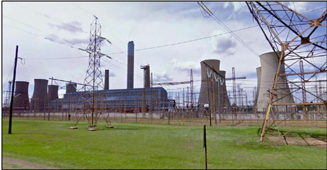
Figure 12: The Komati coal-fired power station and associated infrastructure.
