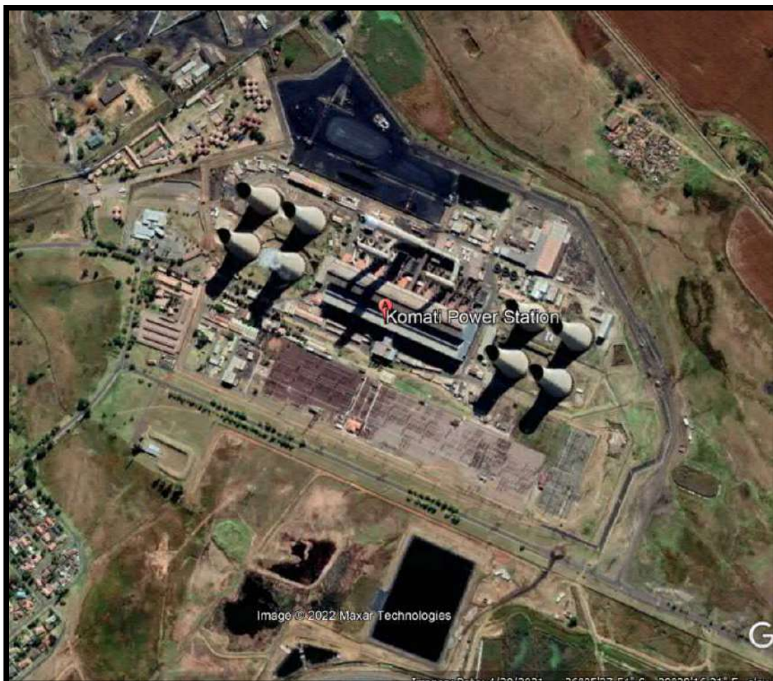
ESKOM KOMATI POWER STATION
