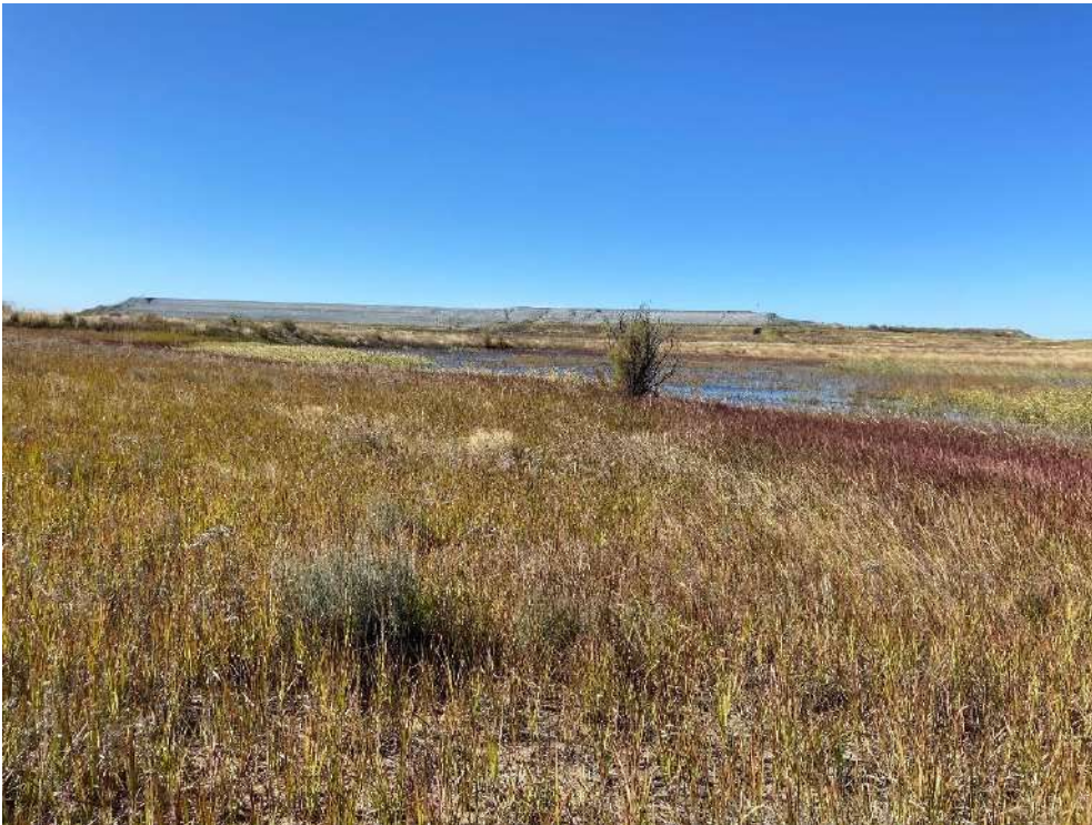
Figure 17: Ash dam facility and pooling of water at dam
