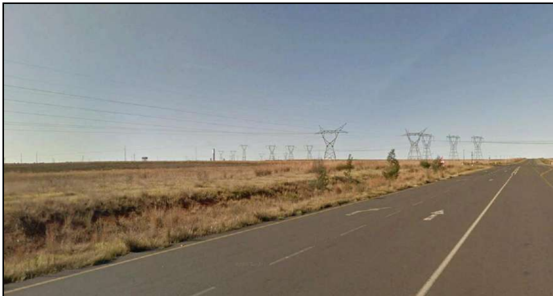
Figure 11: Power lines near the R542 arterial road.
