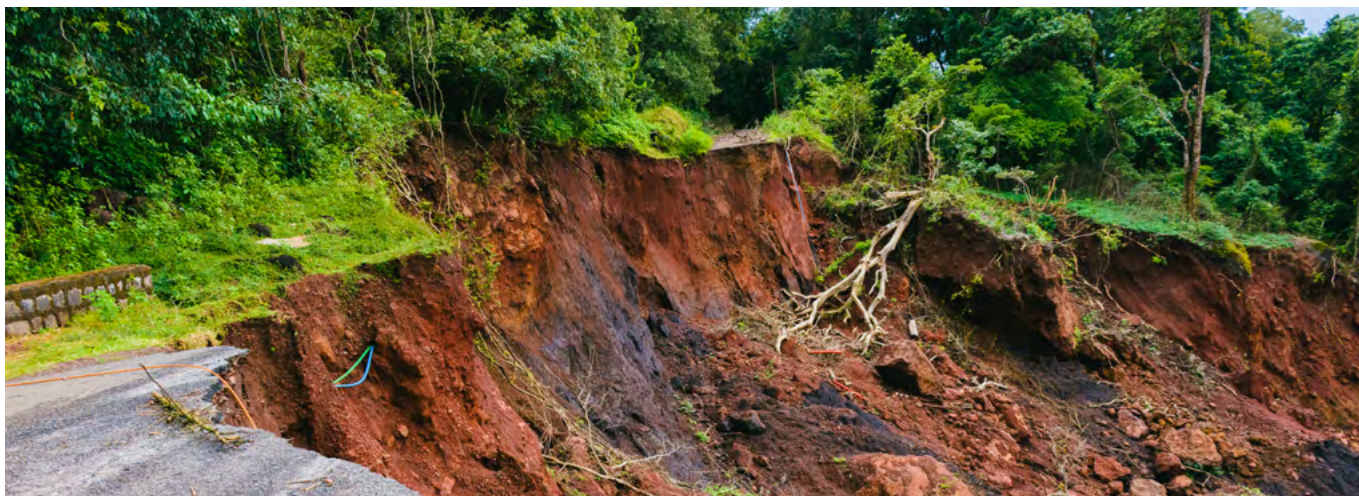
Landslide on a highway in Yellapur, Karnataka, India. © Anwar Attar
