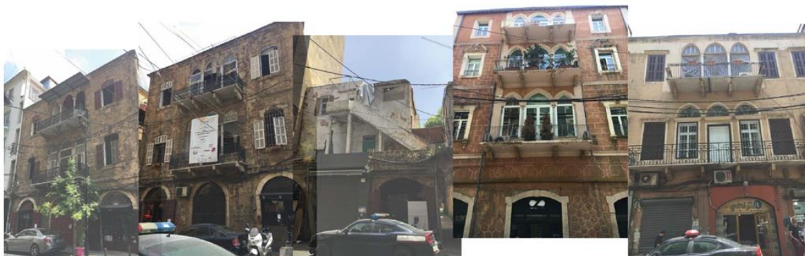
Figure 10. Sample of buildings with heritage value preidentified in the Rmeil and Medawar districts.
