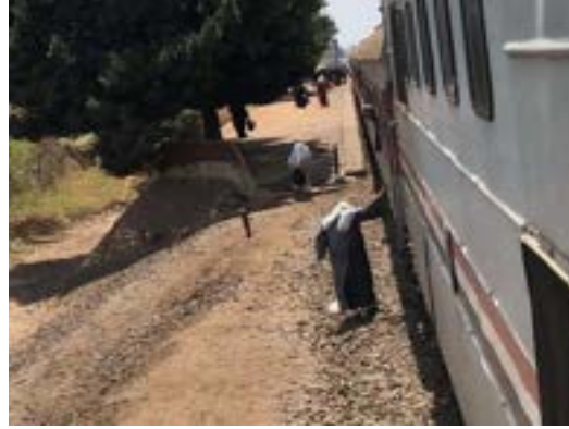
Figure 4-25 Short platform (Al-Akhmas station)
