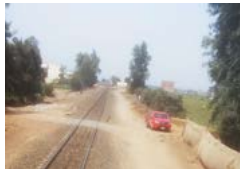
Illegal level crossing and vehicles
