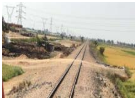
Charcoal kiln and illegal level crossing
