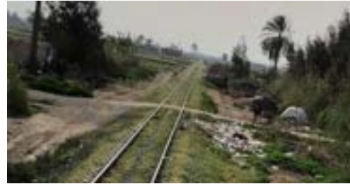
Illegal level crossing and wastes
