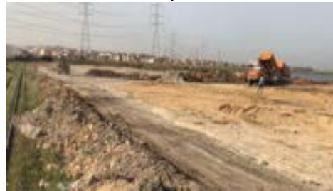
Backfilling of salt pans
