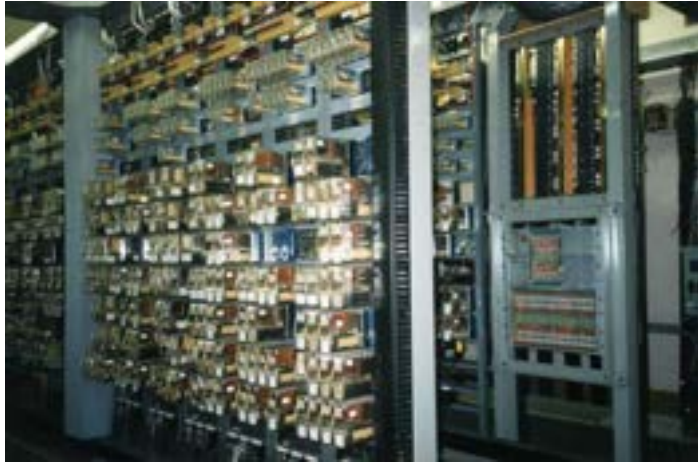
Figure 5-2 Relay interlocking system
