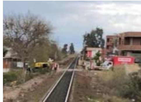
Bad Level crossing
