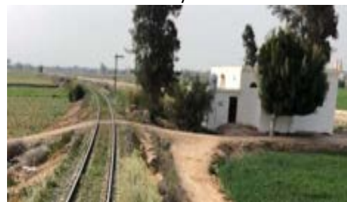
Mosque and illegal level crossing
