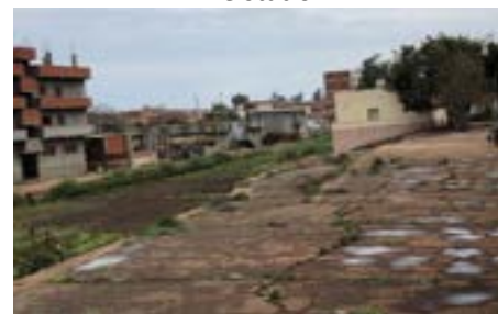
Some houses near the station
