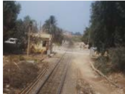
Legal level crossing after the station
