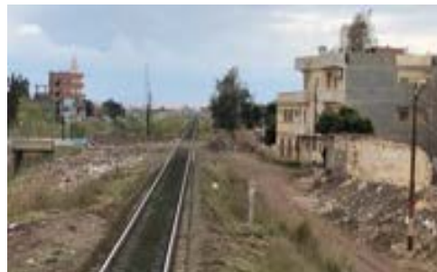
Illegal level crossing and solid wastes
