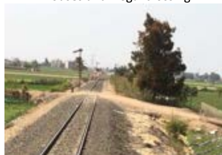
Illegal crossing between agricultural lands
