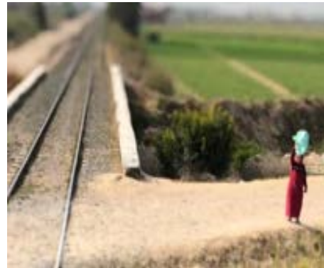
Narrow bridge crosses the watercourse
