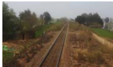
Illegal level crossing for livestock
