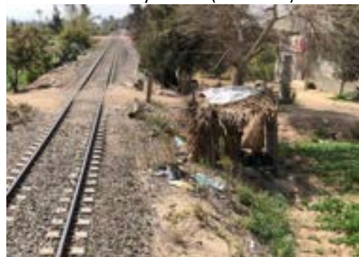
Houses and illegal crossing
