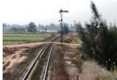
Illegal level crossing between agricultural lands and fish farm
