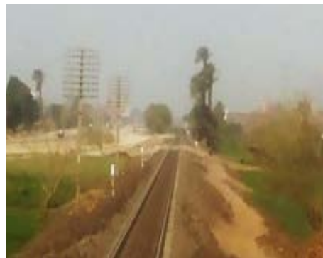
Illegal crossing level
