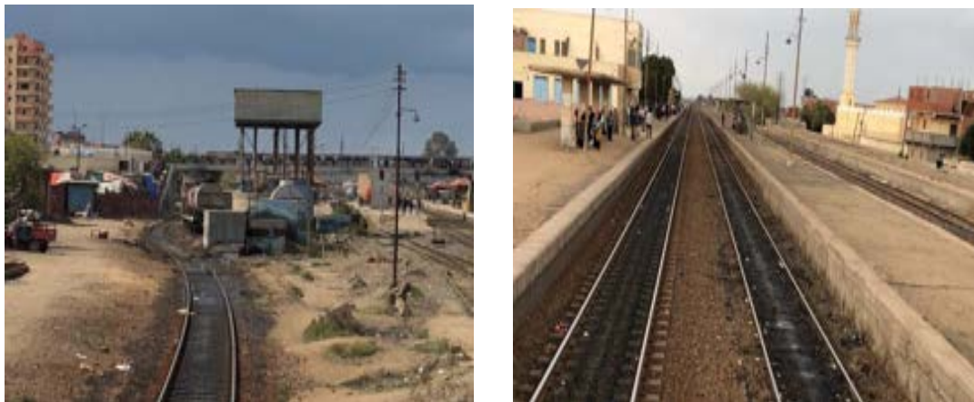
Figure 4-14: Soil Contamination with oil and grease
