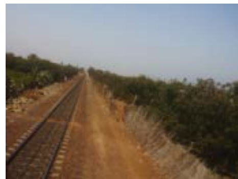
illegal level crossing
