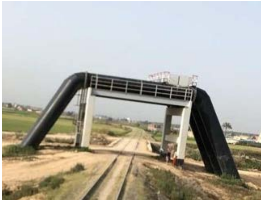
Figure 4-42 Water Pipes in Al-Nahda
