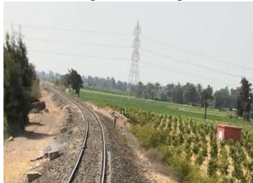
Electricity rooms (both side)
