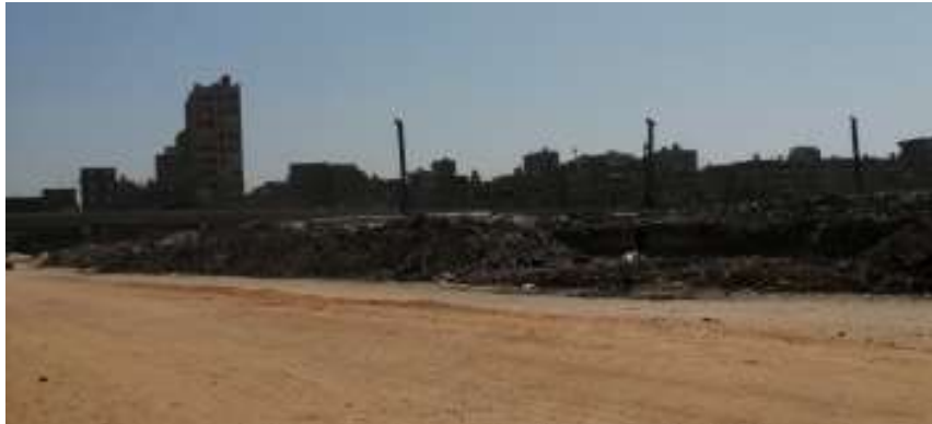
Ring Road expansion works in front of Bashteel station
