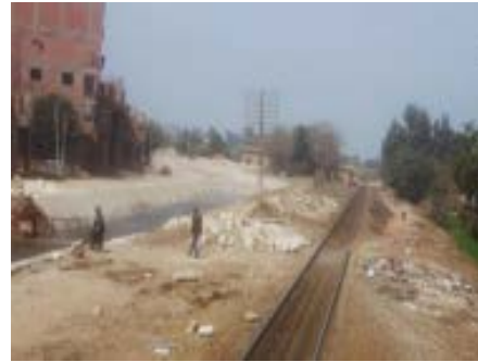
Waste & Pedestrians trespassing on the tracks
