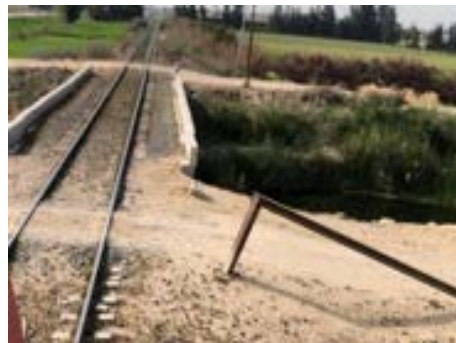
Narrow bridge crosses the watercourse
