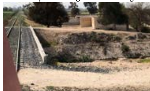
Narrow bridge crosses the watercourse
