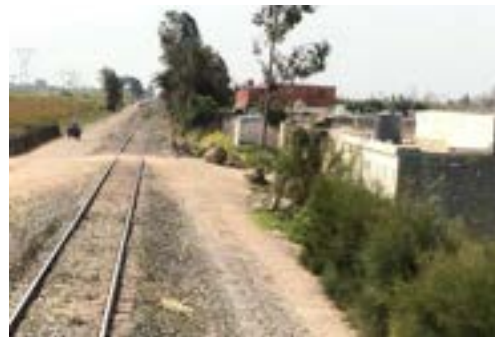
Illegal crossing and houses
