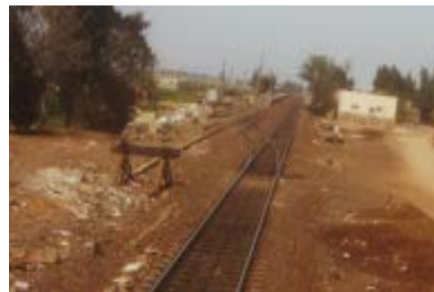
Solid wastes before the station
