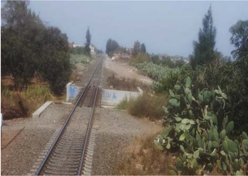
Figure 4-39 train bridge crossing watercourse
