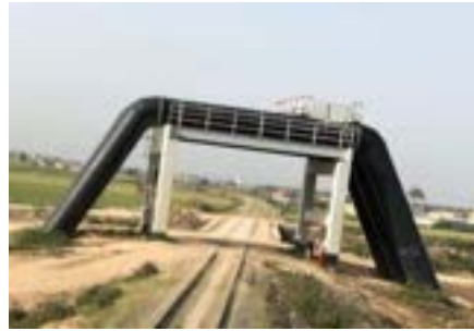
Water Pipes followed by narrow bridge crosses a watercourse
