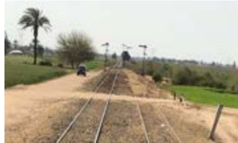
Illegal level crossing and vehicles
