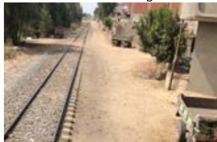
Houses and illegal crossing
