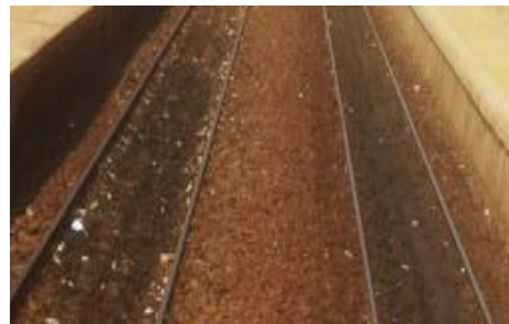
Soil contamination with oil & grease
