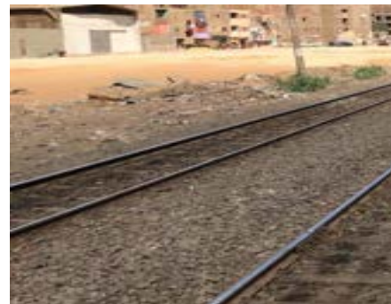
Soil contamination with oil & grease
