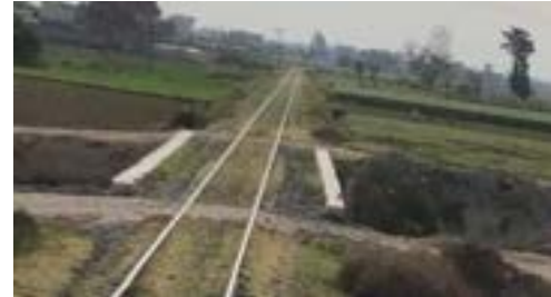
Narrow bridge crosses the watercourse
