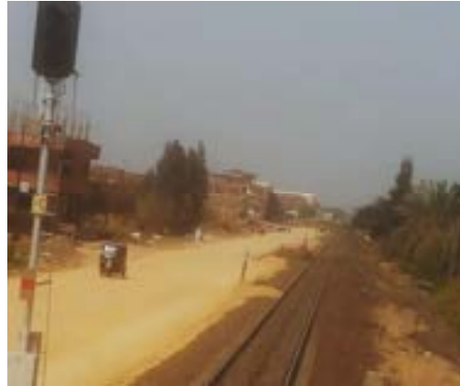
Construction of new road to Sadat.
