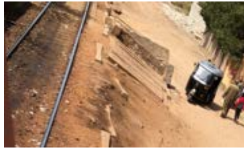
Ramp and Constructed stairs
