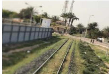
Petroleum company and bad level crossing
