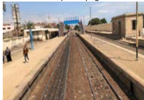
The station and pedestrians bridge
