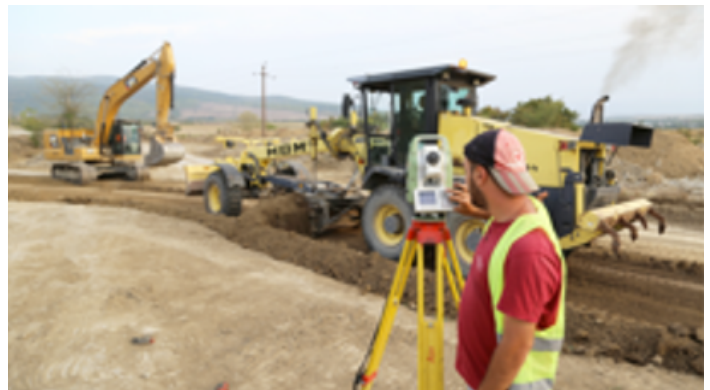
Photo 3.5. Road rehabilitation in the community of Gremiskhevi
