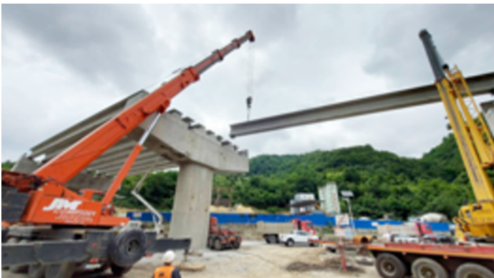
Photo 3.4. Construction of Rikoti Pass Road
