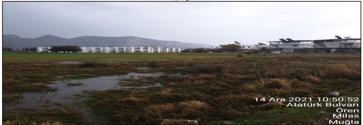
TM-8 Pumping Station
