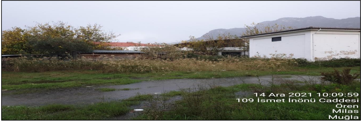
TM-5 Pumping Station
