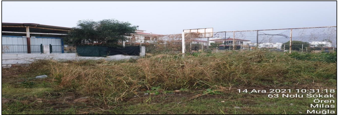
TM-7 Pumping Station
