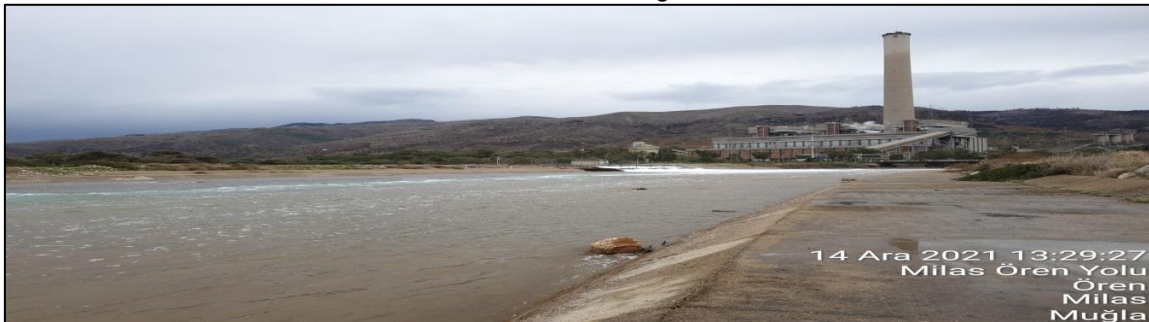
Kemerköy Thermal Power Plant Cooling Water Discharge Located at the Downstream of the Planned Discharge Location
